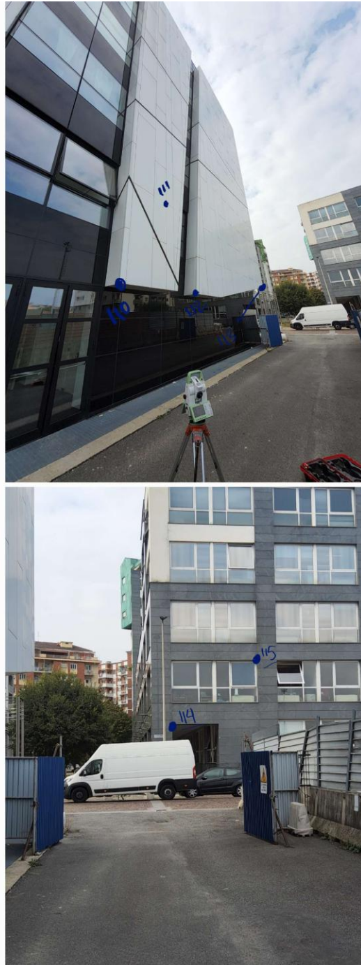
Figure B.7 Exterior control points along the glazed base, with the Total Station in the foreground (top), and further control points along the adjacent street elevation (bottom).
