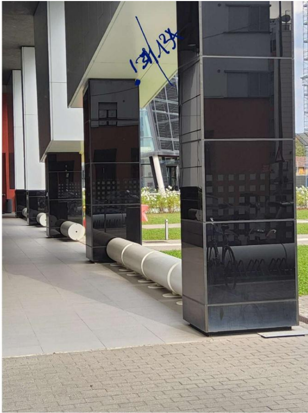
Figure B.8 Instrument orientation notes and exterior control points along the building's angled facade.
