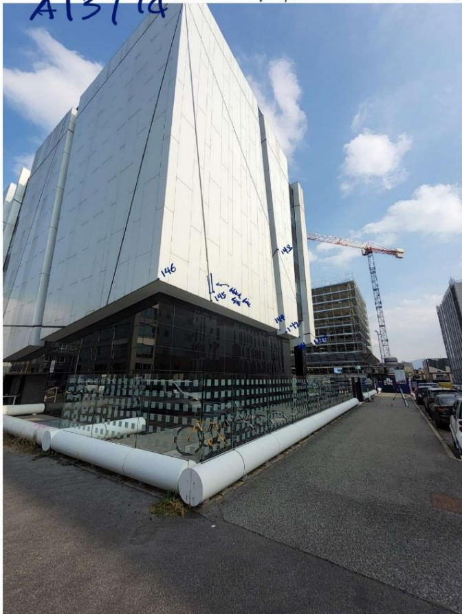
Figure B.9 Total Station setup at point B, oriented to point A, with control points marked along the building's colonnade.
