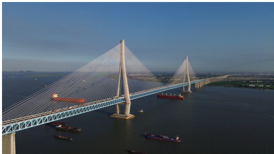
(e) Hutong Yangtze River Bridge
