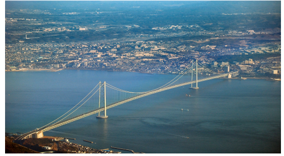
(b) Akashi Kaikyō Bridge
