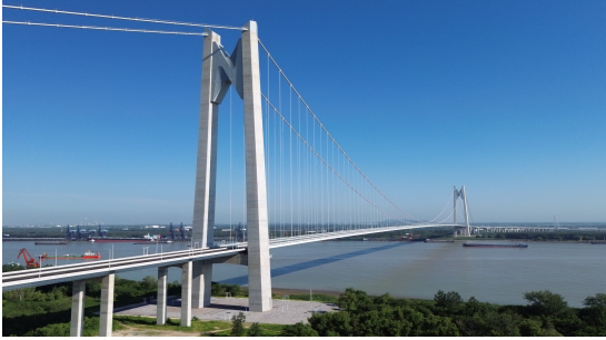
(c) Nanjing Xianxin Yangtze River Bridge
