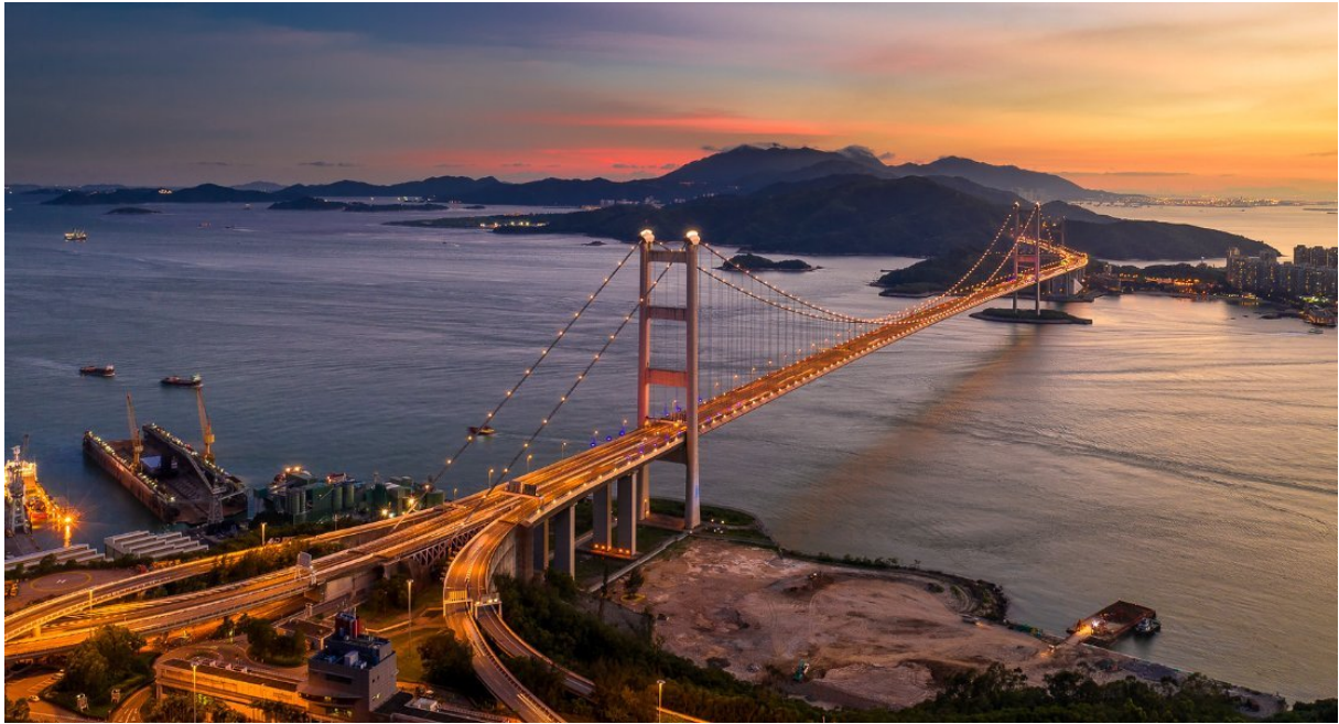
Figure 3.1: Tsing Ma Bridge.
