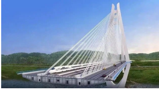
(a) Lingang Yangtze River Bridge
