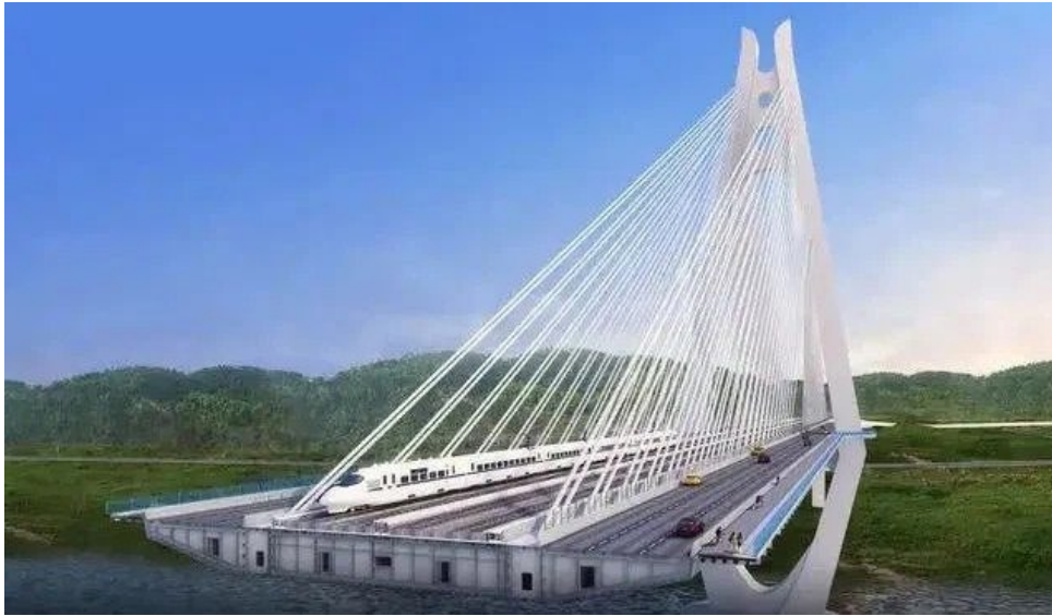
Figure 2.7: Lingang Yangtze River Bridge.
