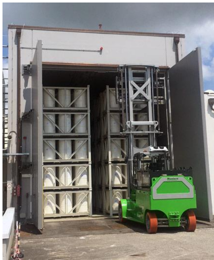
Figure 4.24 Temporary storage facility (Test Tank) at the Trino site
