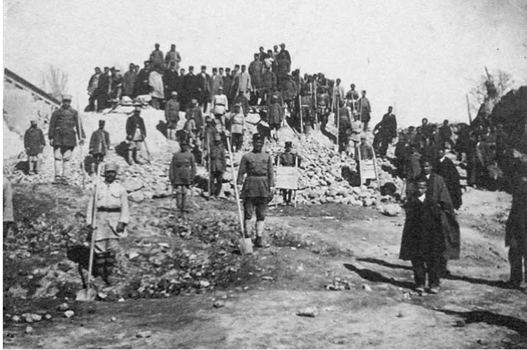
Figure 9: Tarbiat pedestrian crossing during construction. Source: Kojaro
