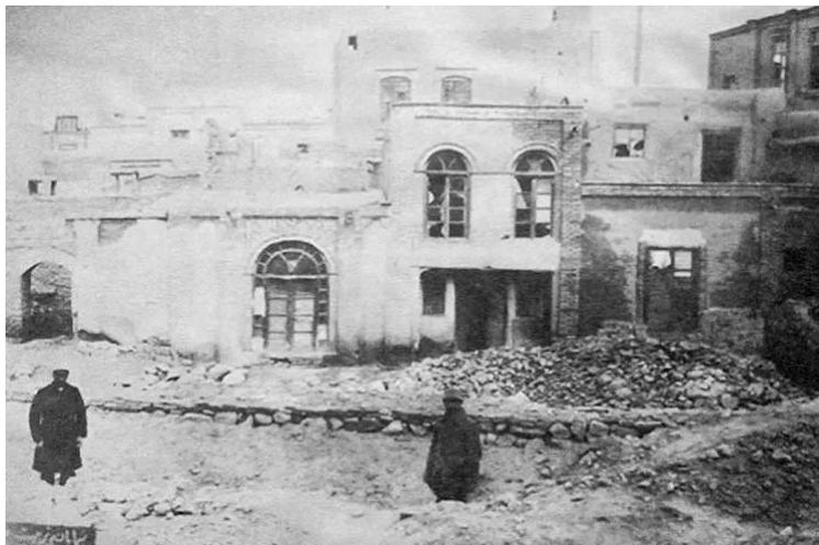
Figure 10: Tarbiat pedestrian crossing during construction. Source: Kojaro
