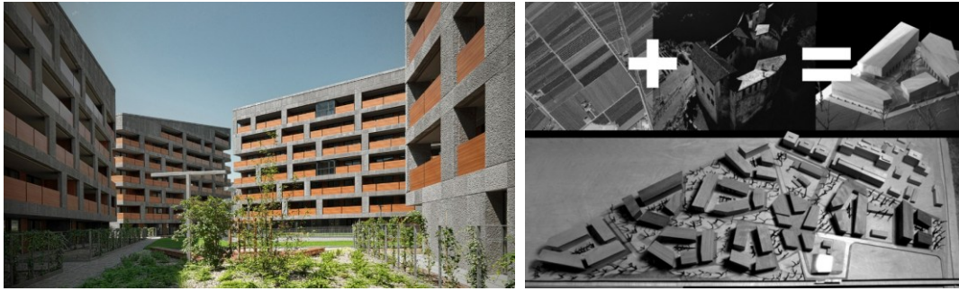
Figure 2.13 Casa Nova eco-community in Bolzano (Source: https://archello.com/project/casanova-masterplan , https://www.archdaily.com/ )
