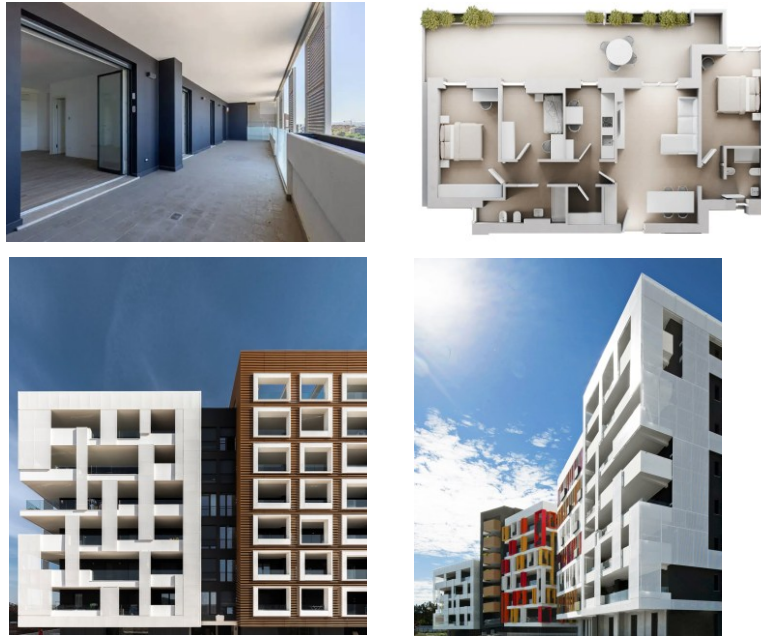
Figure 4.12 The Monti della Breccia project in Rome (Source: https://www.theplan.it/ )
