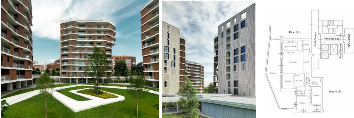
Figure 5.8 Milan, Via Piranesi, 44 (Source: https://www.mabarquitectura.com/ )
