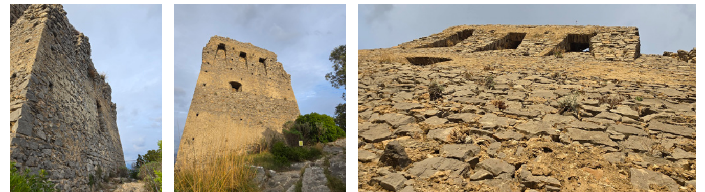
Figure 23 - The actual state of Torre di Montalto. Photographs by the author, acquired October 2nd, 2025
