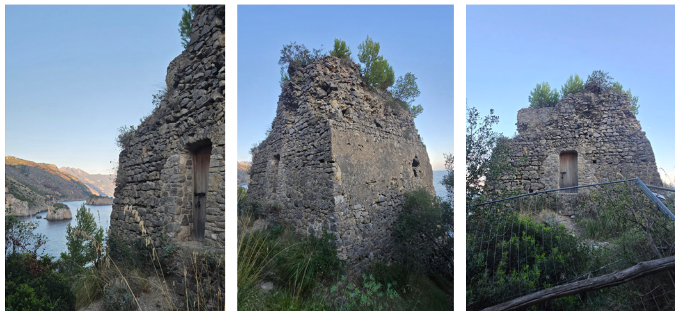
Figure 21 - The actual state of Torre di Recommone. Photographs by the author, acquired September 30th, 2025
