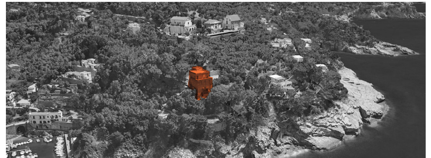
Figure 28 - View of Torre di Capo Corbo. Google Earth Pro satellite image, accessed May 24, 2026.
