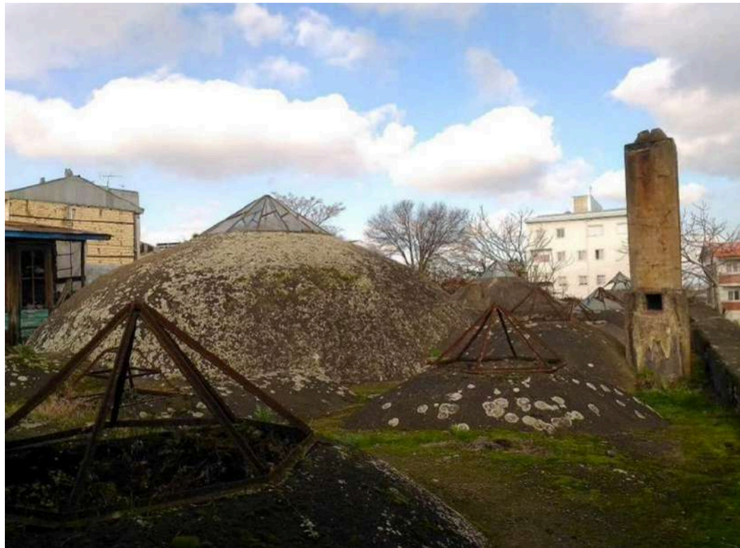
Figure 54- External roof covering of the Haji Bathhouse. Source: Esmailpour Shalamani (2023)
