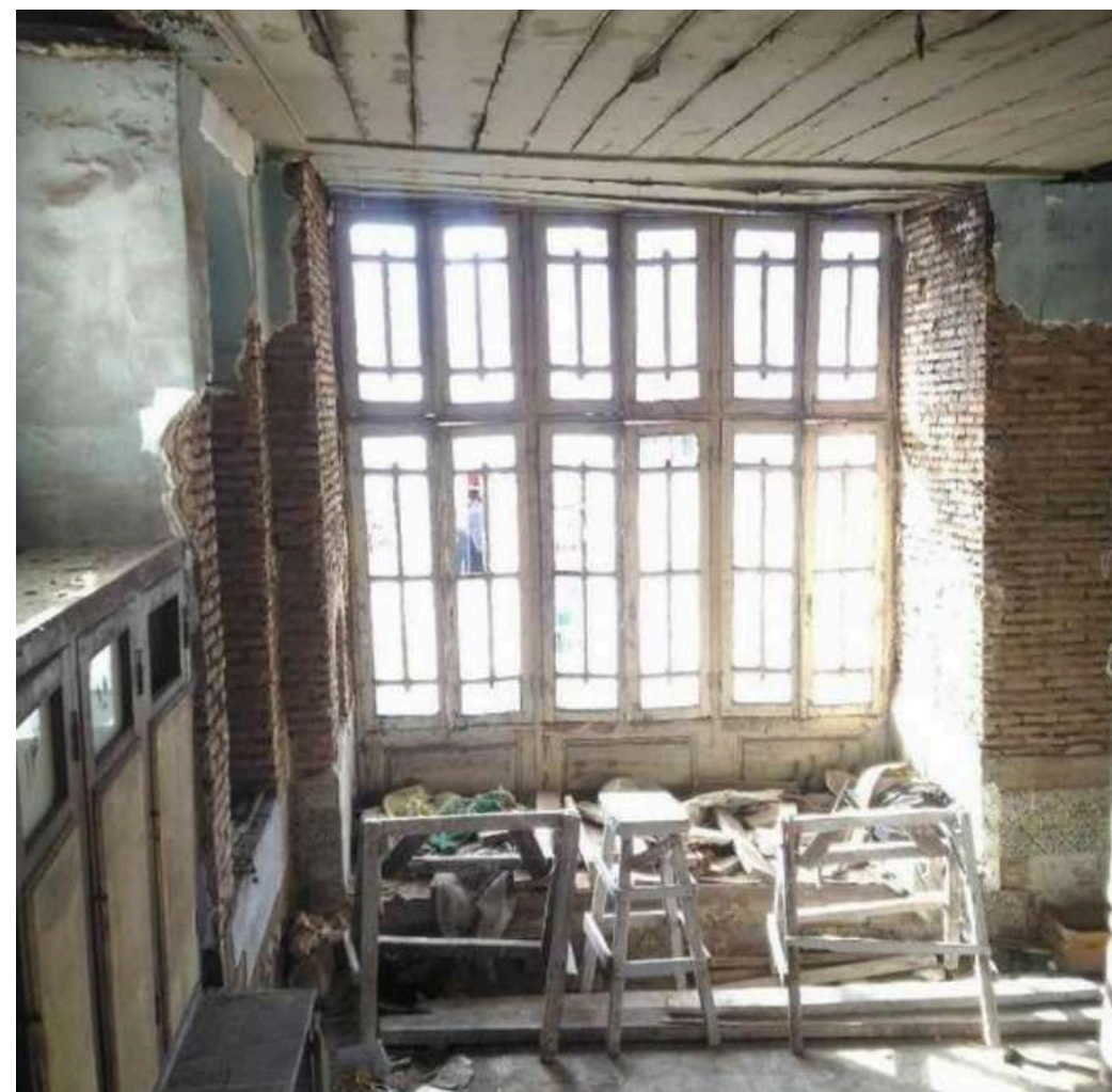
Figure 36-View of the eastern part of the sarbineh from the mezzanine level. Source: Pourghalam Pirbazari (2018).
