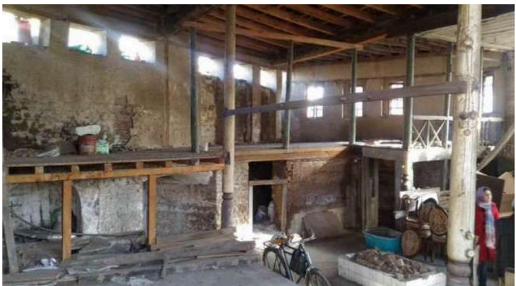
Figure 34- View of the northern part of the sarbineh and the mezzanine level. Source: Pourghalam Pirbazari (2018).
