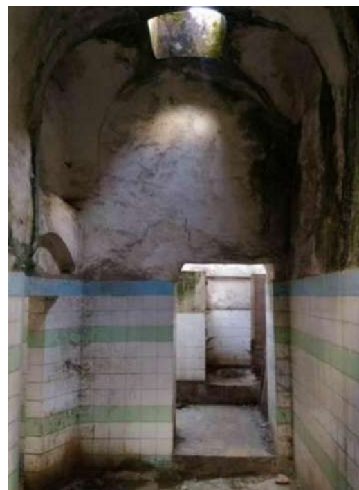
Figure 45- Access to the sanitary facilities from the miyandar. Source: Pourghalam Pirbazari (2018).
