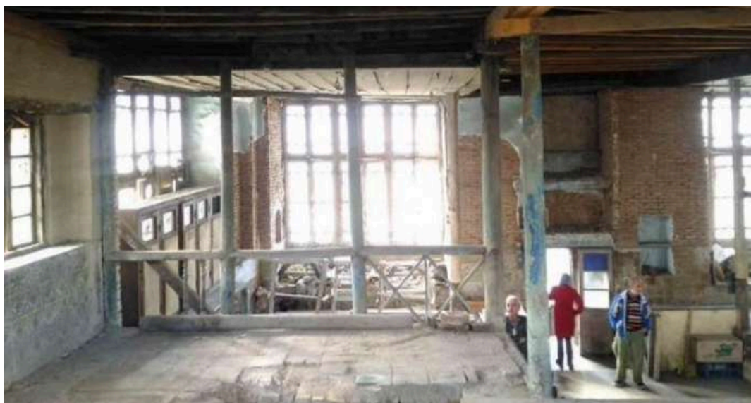
Figure 33- Interior view of the Hajji Bathhouse from the mezzanine level. Source: Pourghalam Pirbazari (2018).
