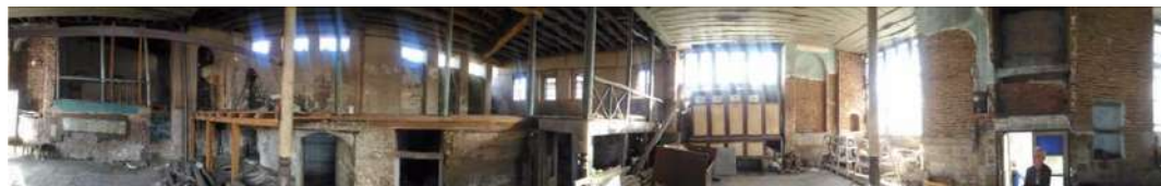
Figure 38- Panoramic views of the sarbineh space in the Hajji Bathhouse. Source: Pourghalam Pirbazari (2018).
