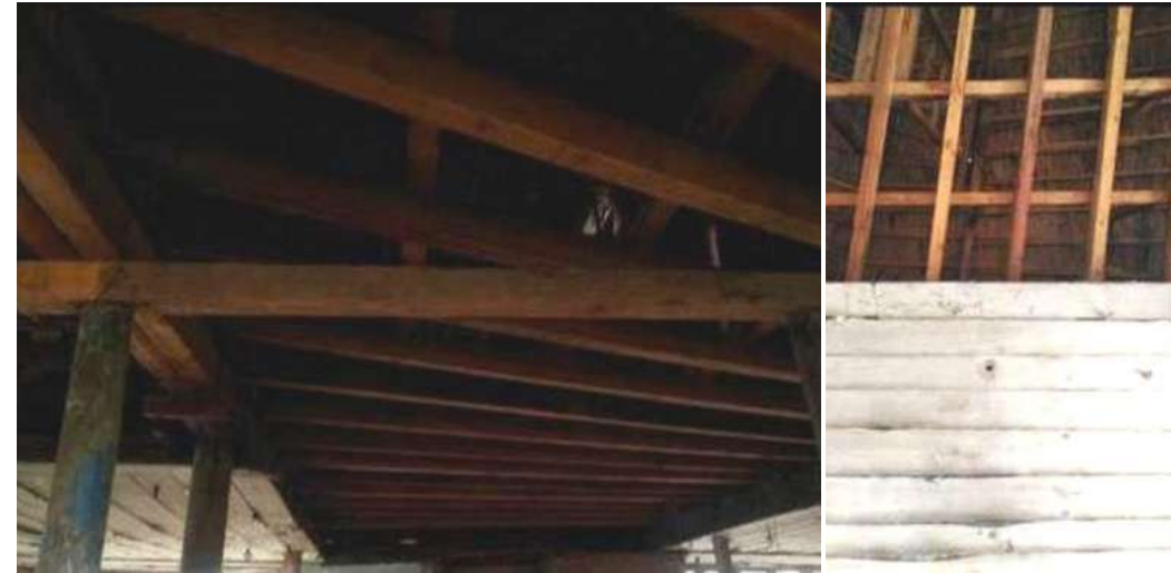
Figure 39- Interior ceiling finish of the sarbineh in the Hajji Bathhouse, showing timber paneling (lambek-kubi). Source: Pourghalam Pirbazari (2018).
