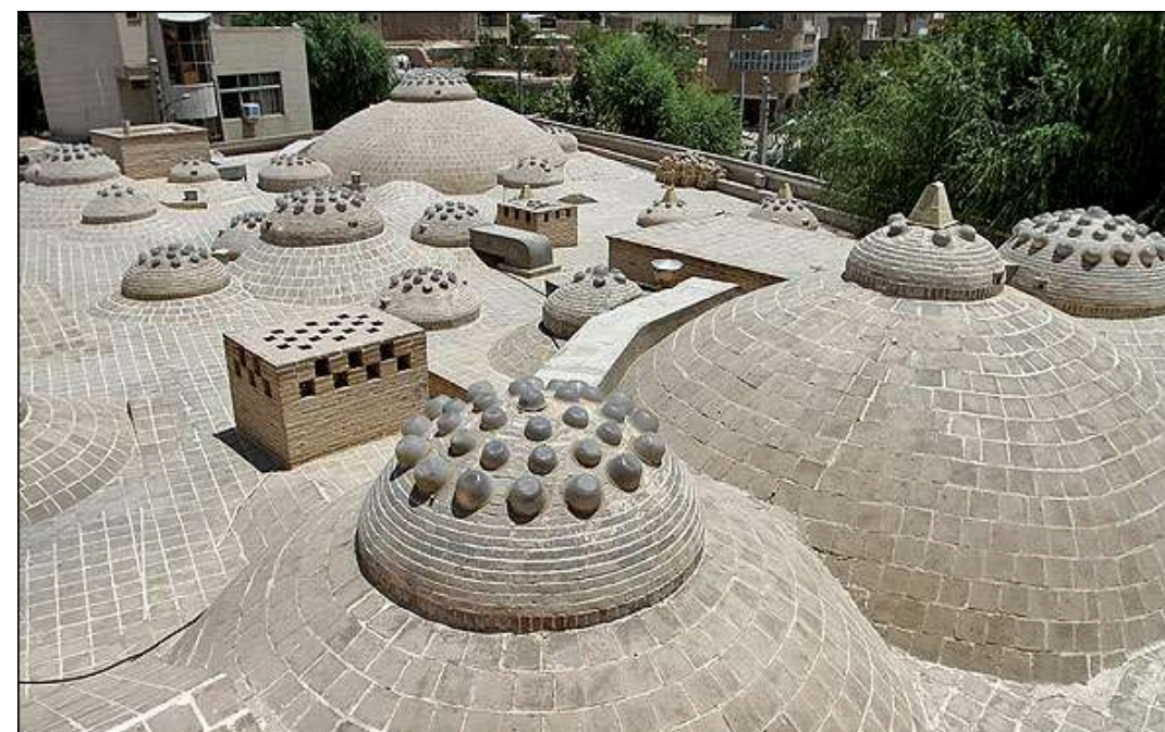
Figure 64- Roof skylights (goljam) of the Ali Gholi Agha Bathhouse. Source: (Kermani, 2017)
