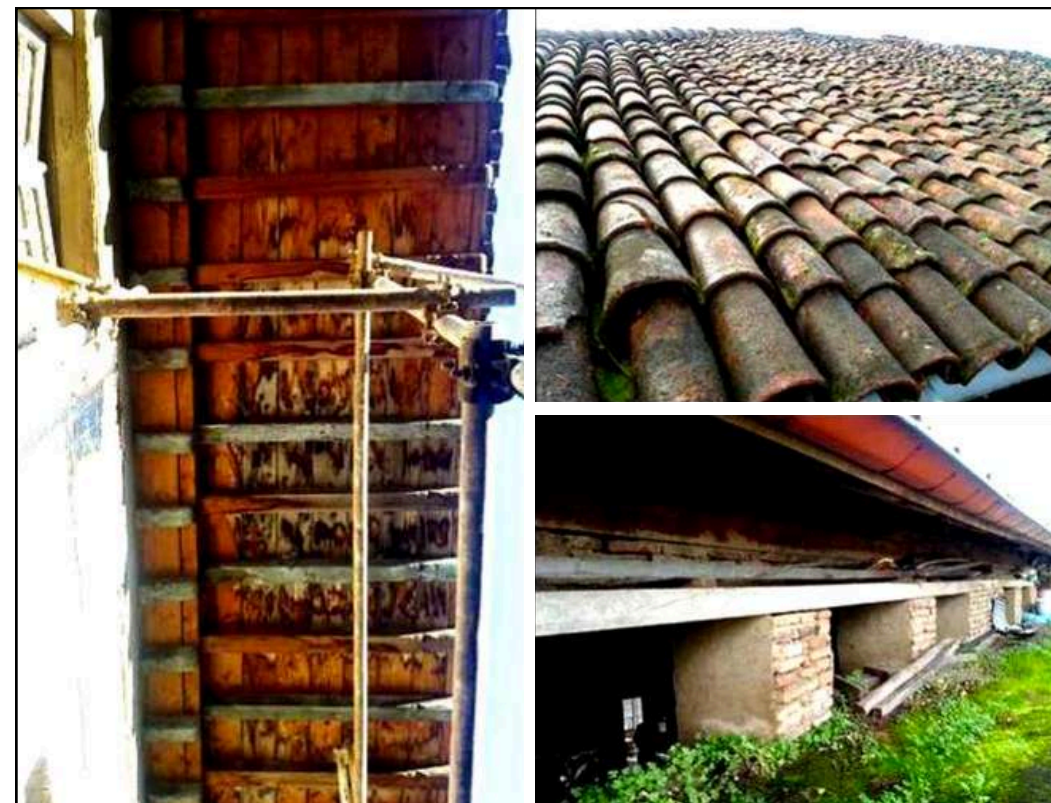
Figure 40- External roof finish of the sarbineh in the Hajji Bathhouse, showing clay tile roofing. Source: Pourghalam Pirbazari (2018).
