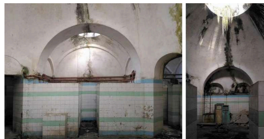
Figure 48- Semi-private bathing chambers. Source: Pourghalam Pirbazari (2018).
