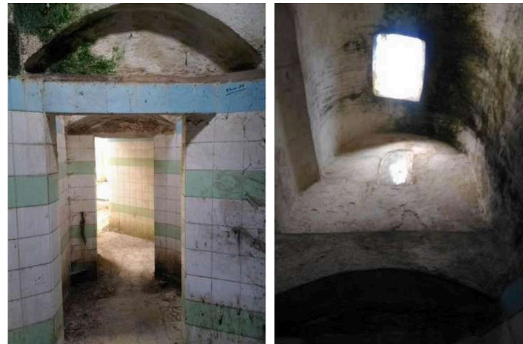
Figure 46- Entrance from the miyandar to the garmkhaneh. Source: Pourghalam Pirbazari (2018).
