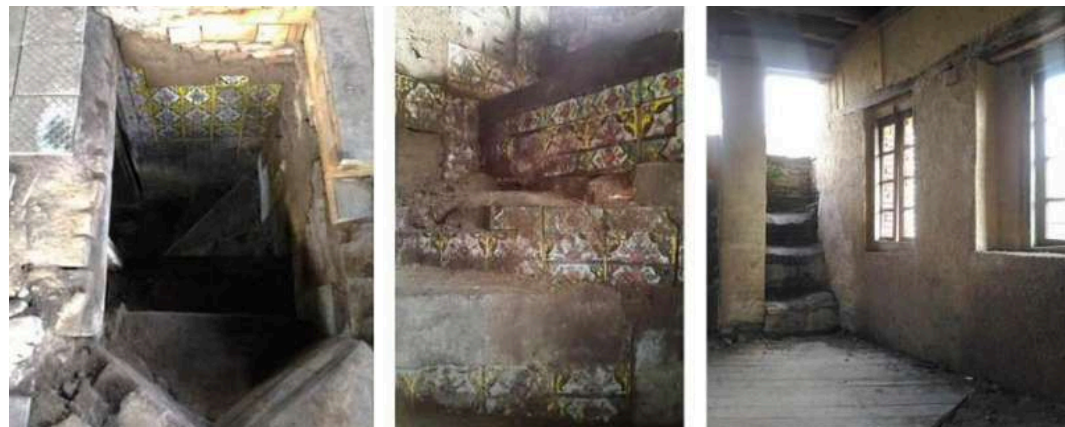
Figure 32- staircase to access to the mezzanine level and roof. Source: Pourghalam Pirbazari (2018).
