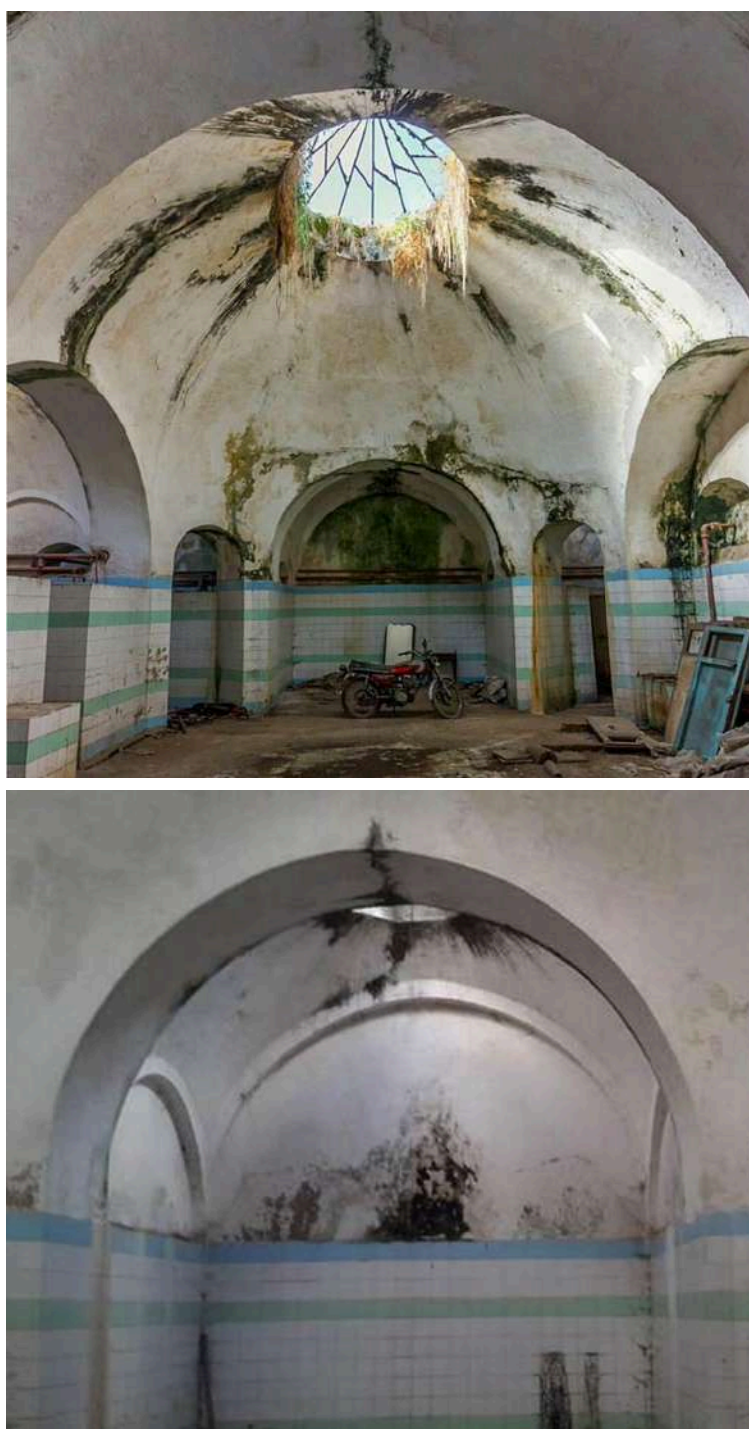
Figure 47- Main dome and central skylight of the hot chamber. Source: Pourghalam Pirbazari (2018).
