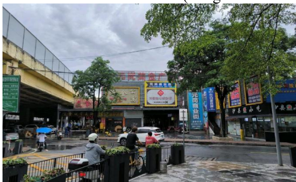
a) Before Renovation
