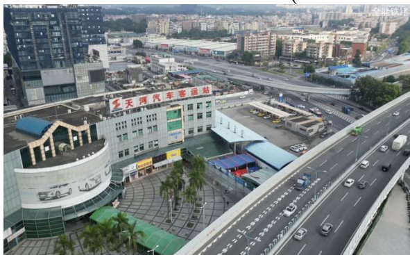
a) Before Renovation
