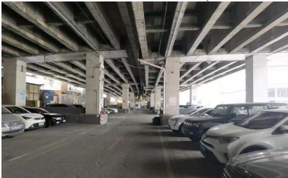
a) Before Renovation
