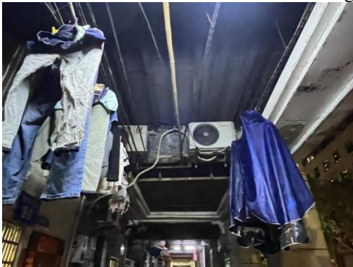
Clothes Drying, External Air-Conditioning Units
