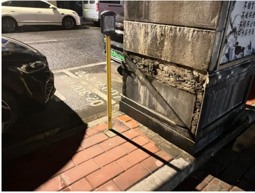
Raised Platform Installations
