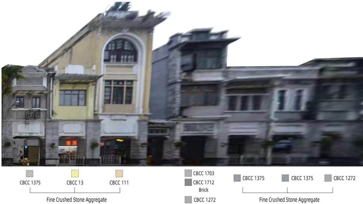
Figure 6-15 Original Facade Of The Key Area — East Side
