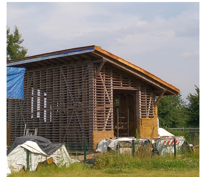
Figure 3.9: Experimental construction processes at the Grugliasco site, illustrating student participation in the assembly of bio-based building systems
