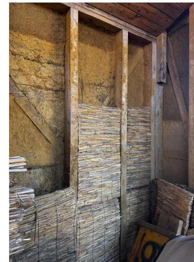
Figure 3.3: A photo of a wall build-up in one of the Experimental Pavilions (Grugliasco) showing the assembly of bio-based building materials ( straw, hemp, timber, earth) layered as a wall element.
