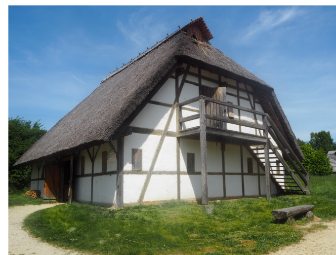
Figure 2.7: A house made from clay bricks, clay rendered walls, timber and straw. Source: Naturdorf Bärnau photo archive
