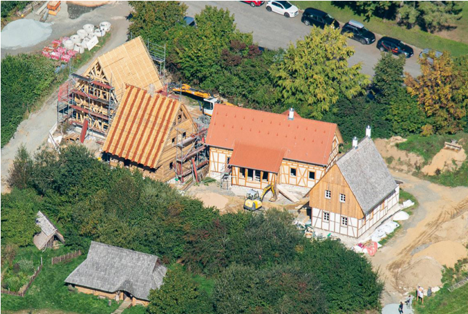
Figure 2.13: The Naturdorf holiday homes under construction shows diverse use of materials (Labelled A-D from left to right. Source: Naturdorf Bärnau photo archive. https://www.naturdorfbaernau.de/
