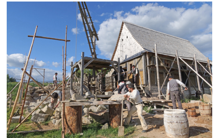
Figure 3.4: Construction process of the Royal court on a demonstration site next to the Bärnau History Park with craftsmen using medieval techniques and tools to erect a stone building complex. Photo by: Geschichtspark Bärnau-Tachov
