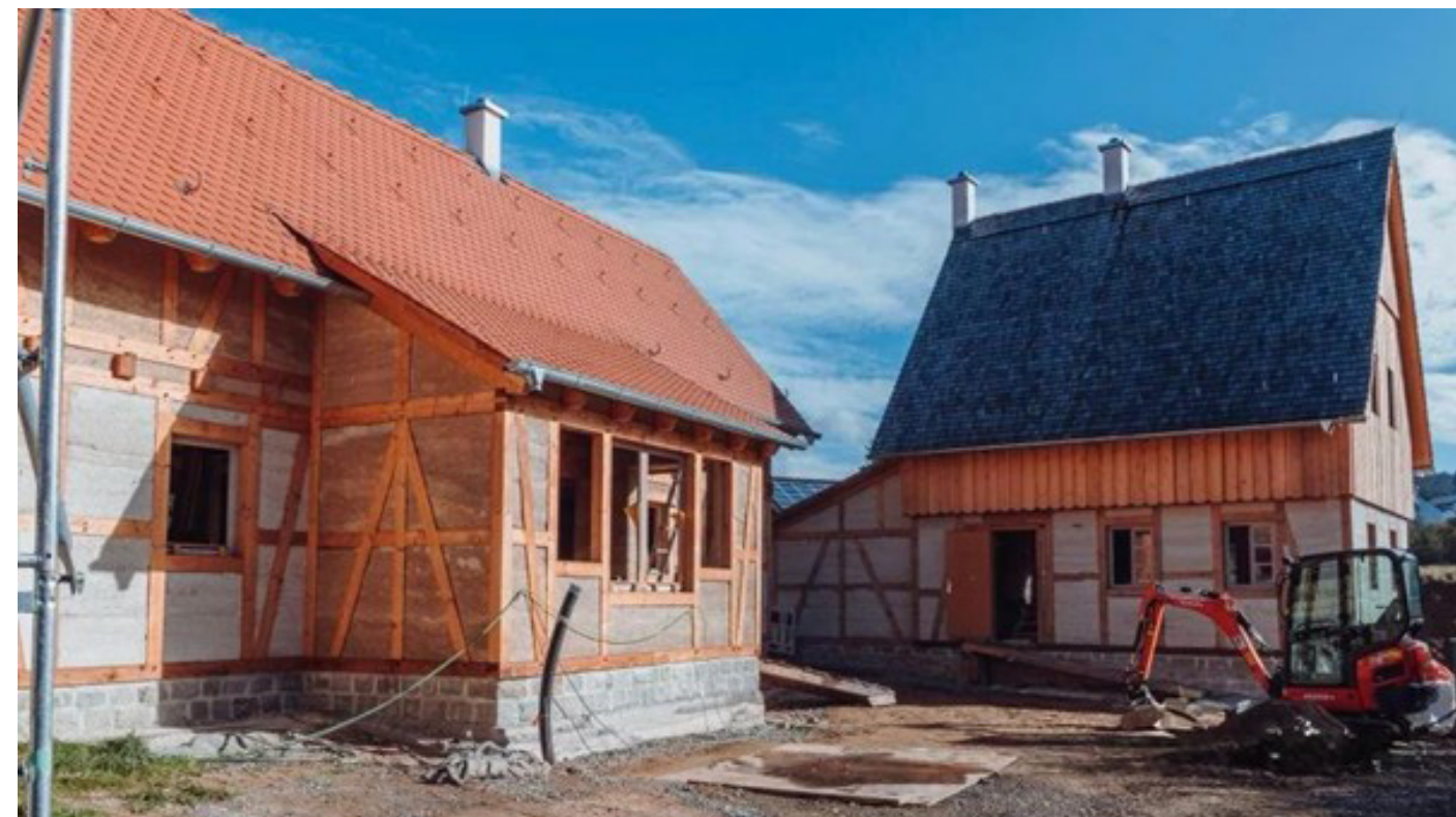
Figure 2.14: Houses C and D of the Naturdorf under construction (Building C and D on the left and right respectively). Sourced from Onetz.de photo archive
