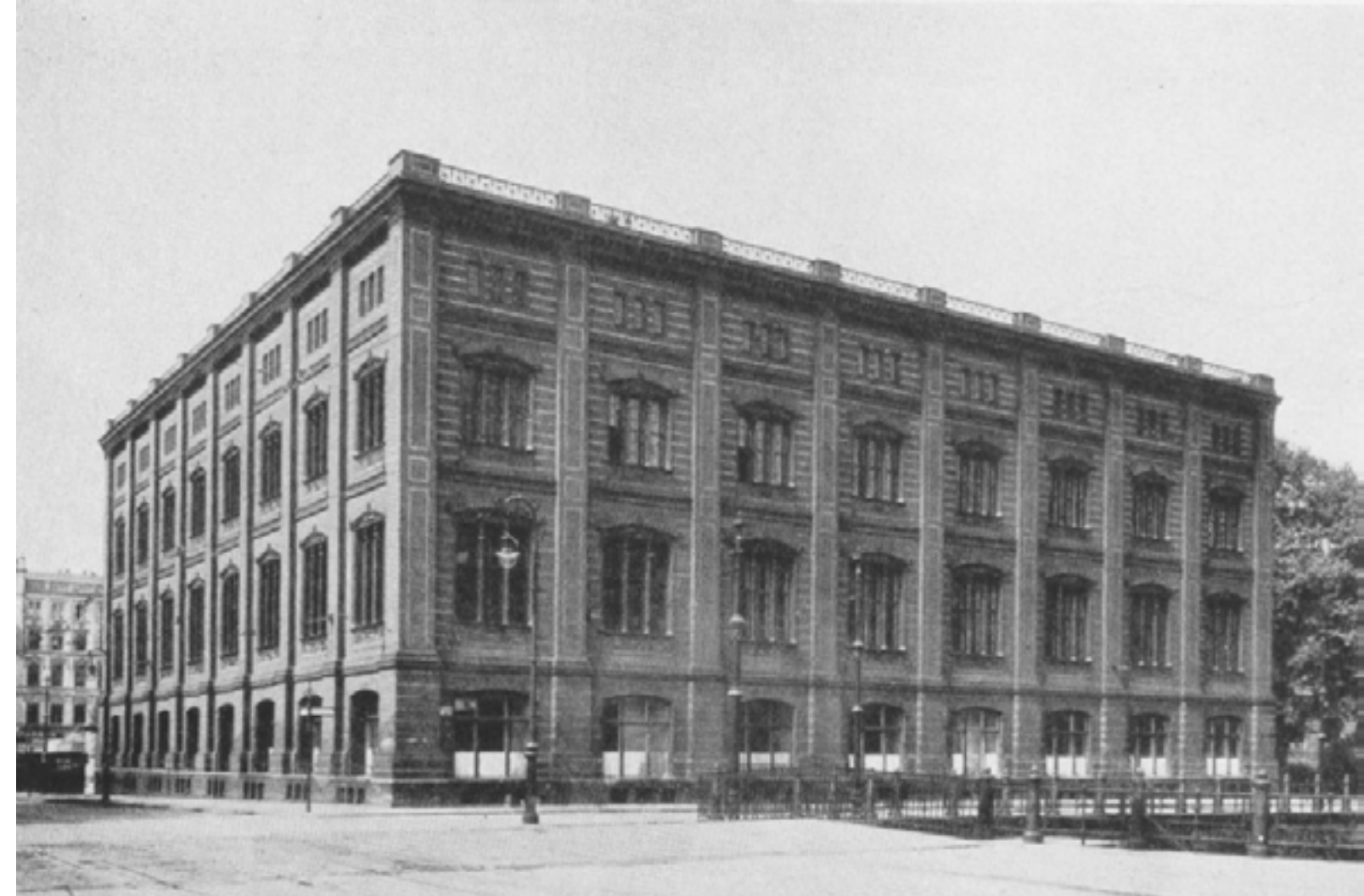
D.58. Berlin, Bauakademie | Historical photo
