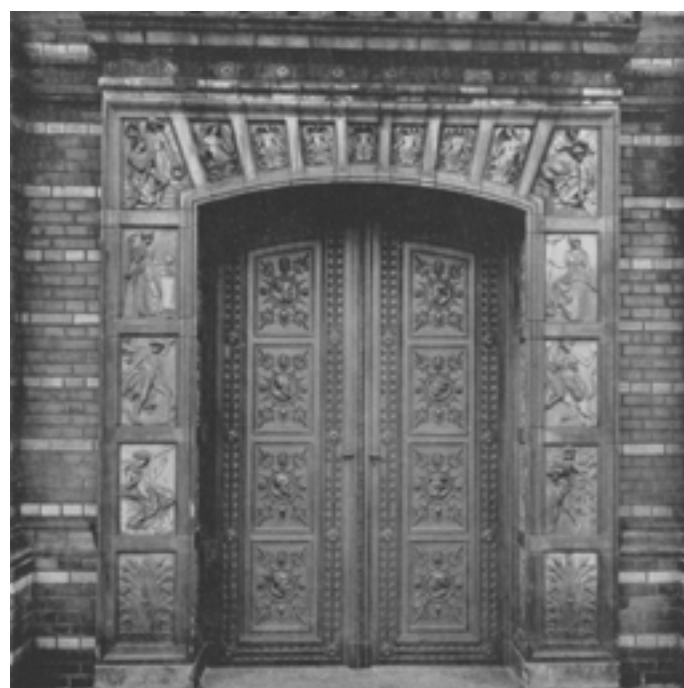
D.53. Berliner Bauakademie | Portal | 1911
