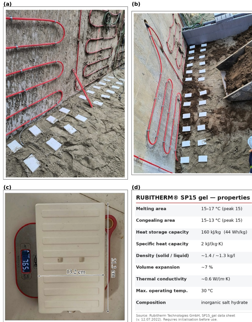
Figure 12: Macro-encapsulated PCM (Rubitherm® SP15 gel) installed in field 1: (a, b) tab distribution on the ground in front of the energy wall during backfilling; (c) single tab, 13.2 × 21.3 cm, 765 g; (d) main material properties (Rubitherm SP15_gel data sheet), after Alvi (2026).
