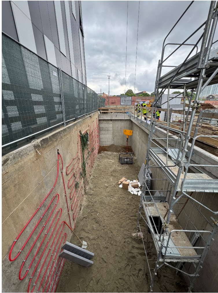
Figure 10: Upgraded geothermal wall with 6 circuits during construction
