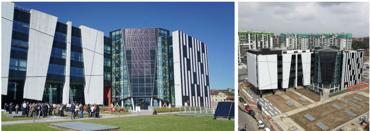
Figure 3: Exterior views of the Energy Center building at Politecnico di Torino, where the Geothermskin experimental prototype is installed on the underground retaining wall
