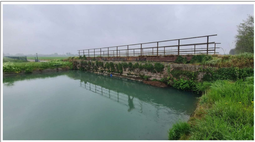
Image 3.4 – Lateral view of a crossing work on the Cavour canal characterized by the presence of a continuous structure in concrete and by a simple metal railing. The image highlights how the support structure of the bridge enters directly into contact with the free surface of the current, which notably alters the stationary structure of the flow.
