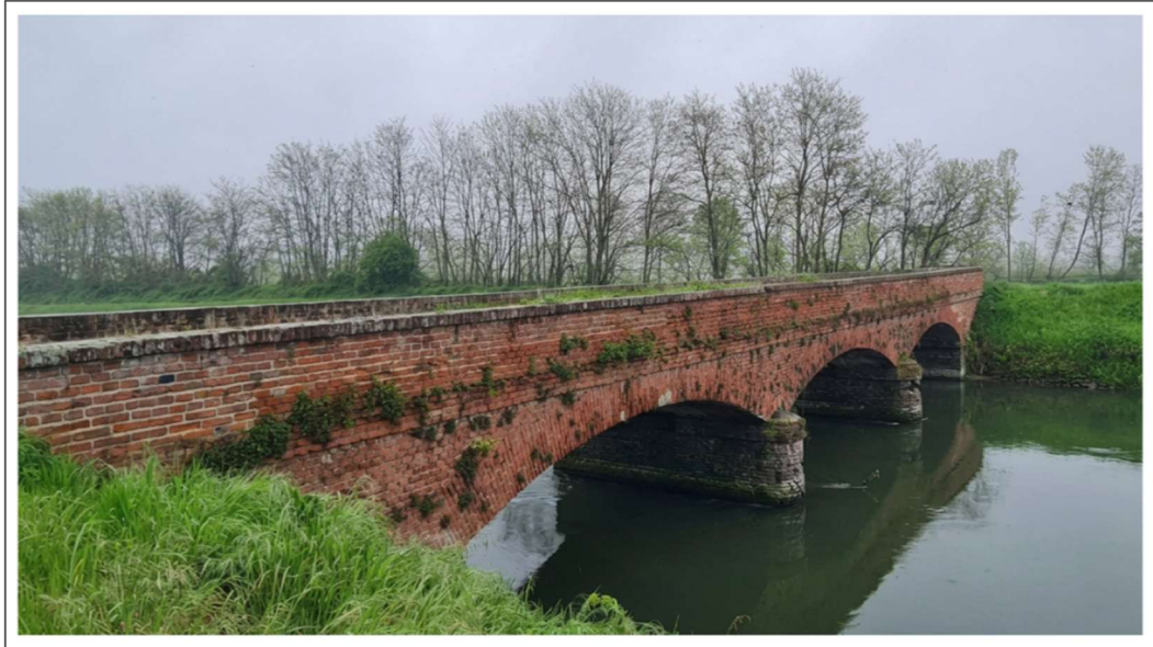
Image 3.3 – Lateral view of a historical brick arch bridge that crosses the canal, for the crossing of the Cavour canal. From the present image is clearly evident the dimension of these structures that impose constraints of a logistic type: the enormous structure does not offer easy or safe anchor points for the rigid fixing of the instrumentation for the acoustic profiling.
