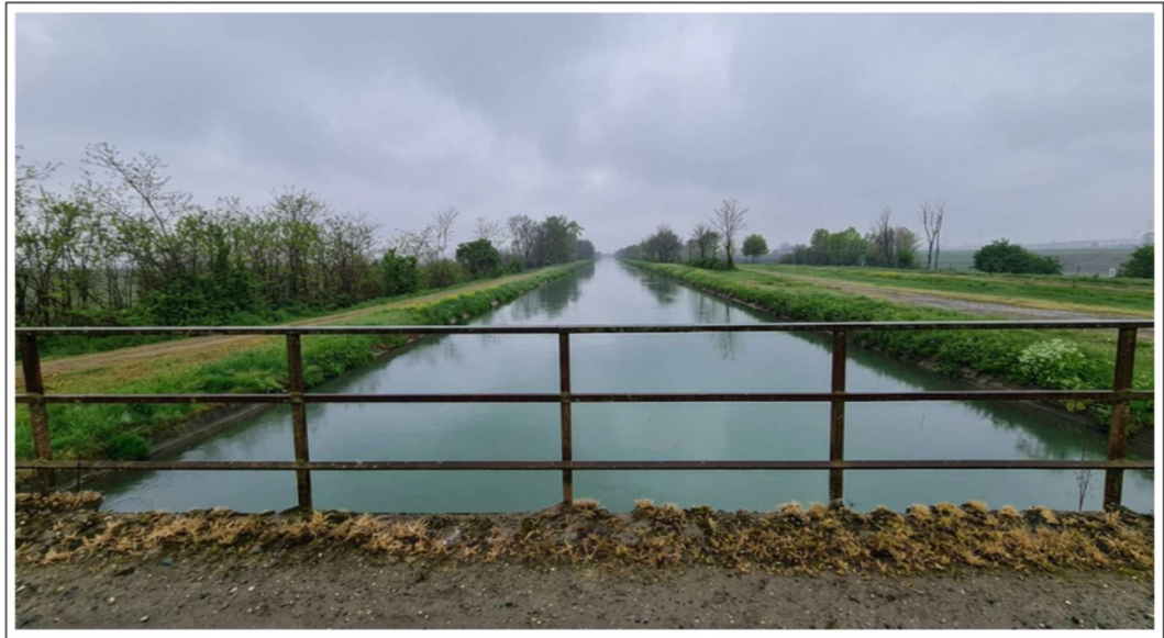
Image 3.1 – View of the Cavour canal taken from the centerline of a pedestrian bridge, which highlights the notable linearity of the stretch towards upstream, with respect to the direction of the water flow, and the wide cross-section of the canal. Although such uninterrupted geometric regularity initially seemed ideal for the purpose of sampling velocity time series, evidence gathered in the field revealed the presence 50 meters further downstream of a water intake directed towards a secondary parallel branch.
