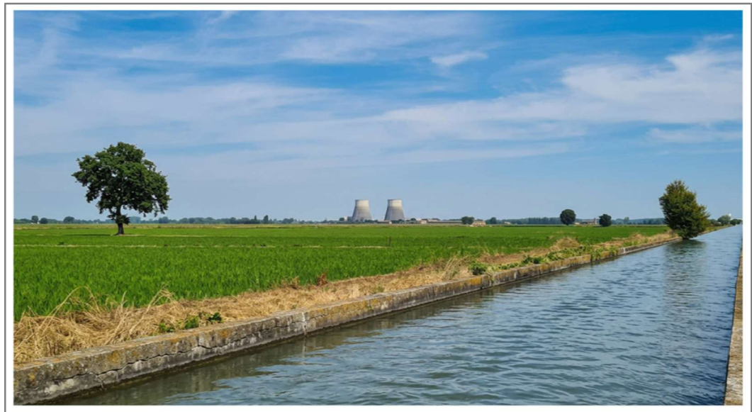
Image 3.7 – Photographic image of the Cavo Lucca taken during the inspection in the field, which highlights the linearity of the stretch upstream of the sampling section. The image clearly evidences the geometric regularity of the irrigation canal, with the flow delimited by extremely regular vertical concrete banks and characterized by the absence of intrusive vegetation in direct contact with the free surface of the water.
