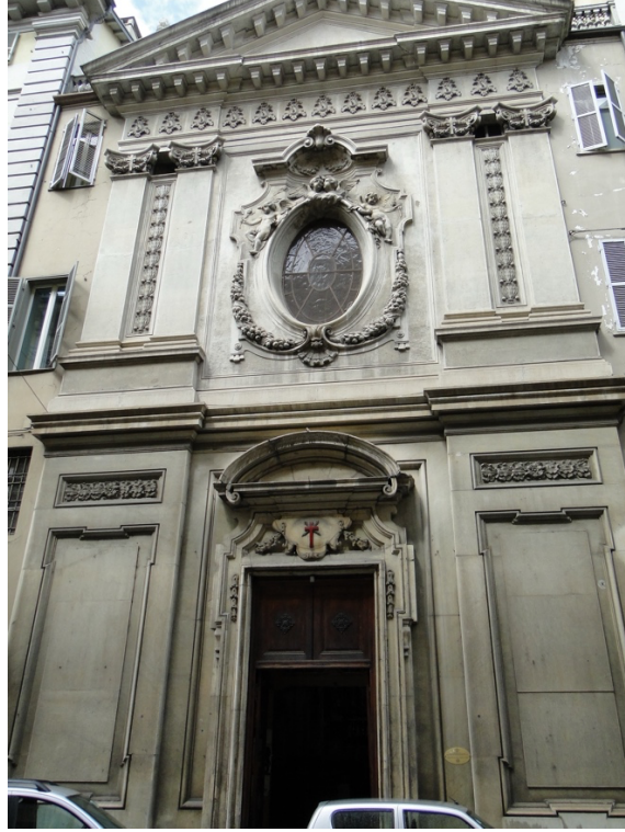
Figure 1. Facade of the church of San Giuseppe
