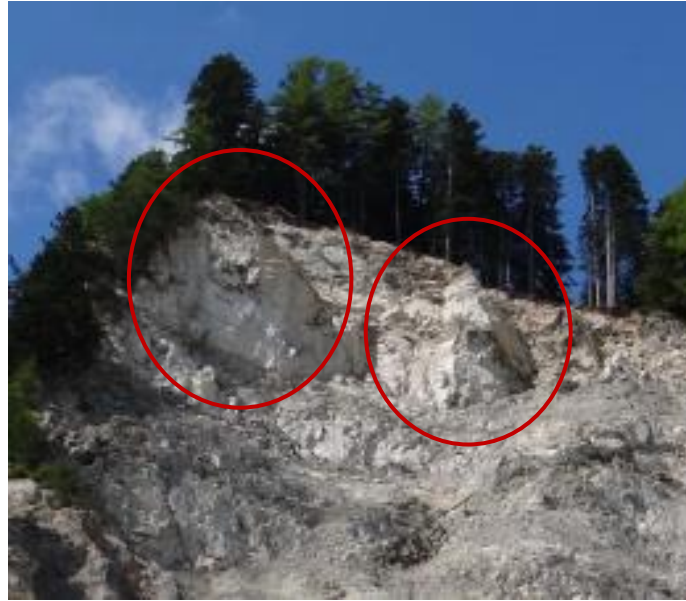
Figure 7: Zoom on the Gollone landslide at the 29 may 2012. From ARPA Piemonte, SIFraP report, 2013
