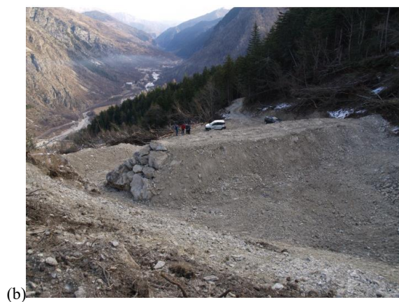
Figure 9: (a) Protection systems map, map produced in QGIS (b) Embankment realised after the landslide of 2011, picture taken the 29 December 2011 and linked to SiFraP report 2024.
