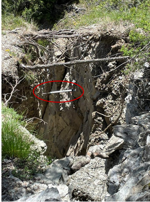
Figure 11: Wire extensometer installed by ARPA Piemonte in 2021. Image taken on the 28 May 2024.
