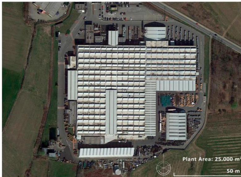
Figure 28 Aerial satellite view of the industrial plant site, highlighting the 25,000 m 2 rooftop footprint evaluated for the photovoltaic retrofit installation.
