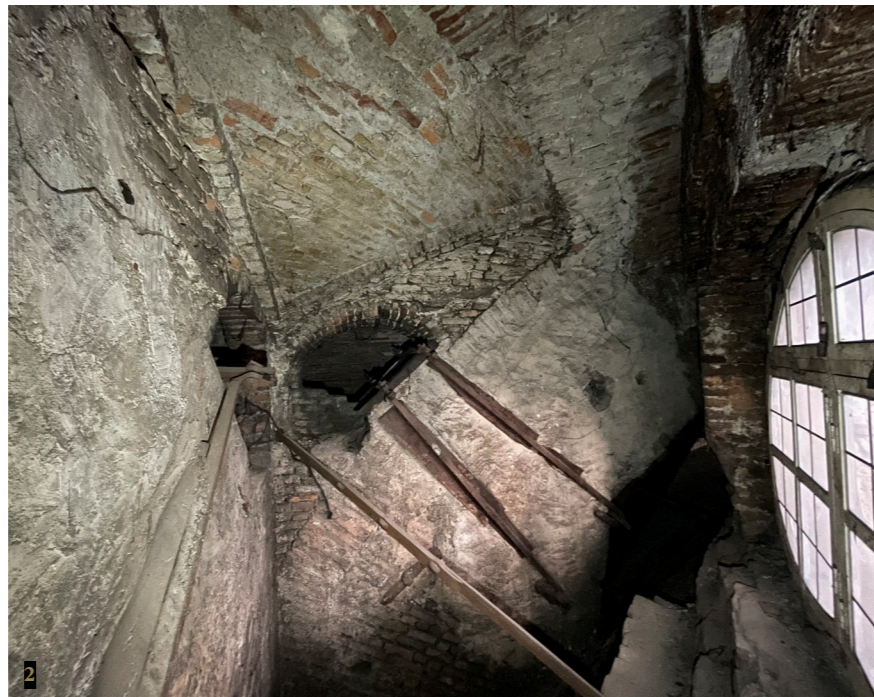
Corner tower's opening, and the springing of the arconi on the left.
