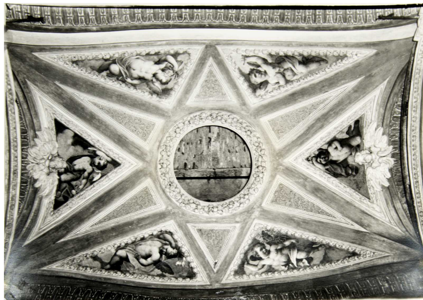
Figure 53— The star-shaped vault. From Fondo Passanti
