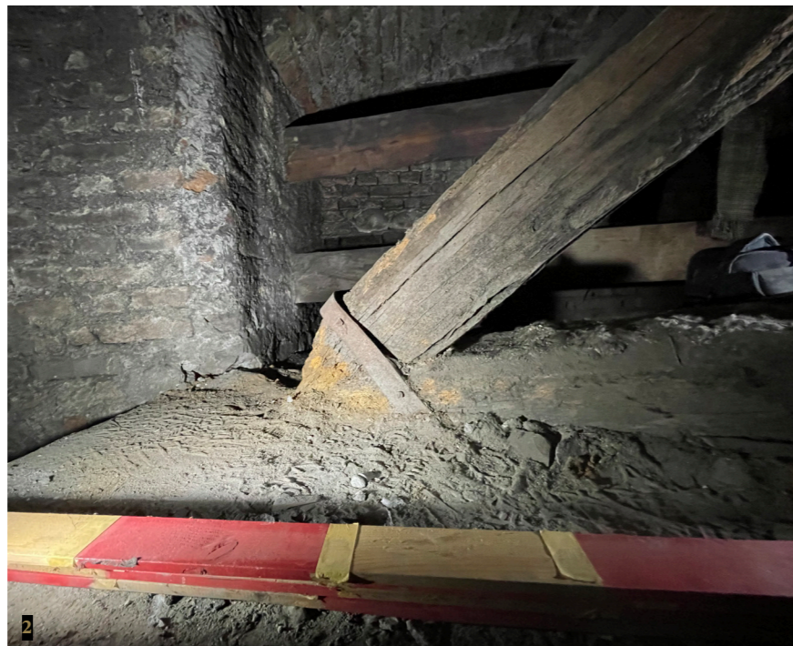
Chiave della Cupola's interaction with Randoni's additional vault to walk on
