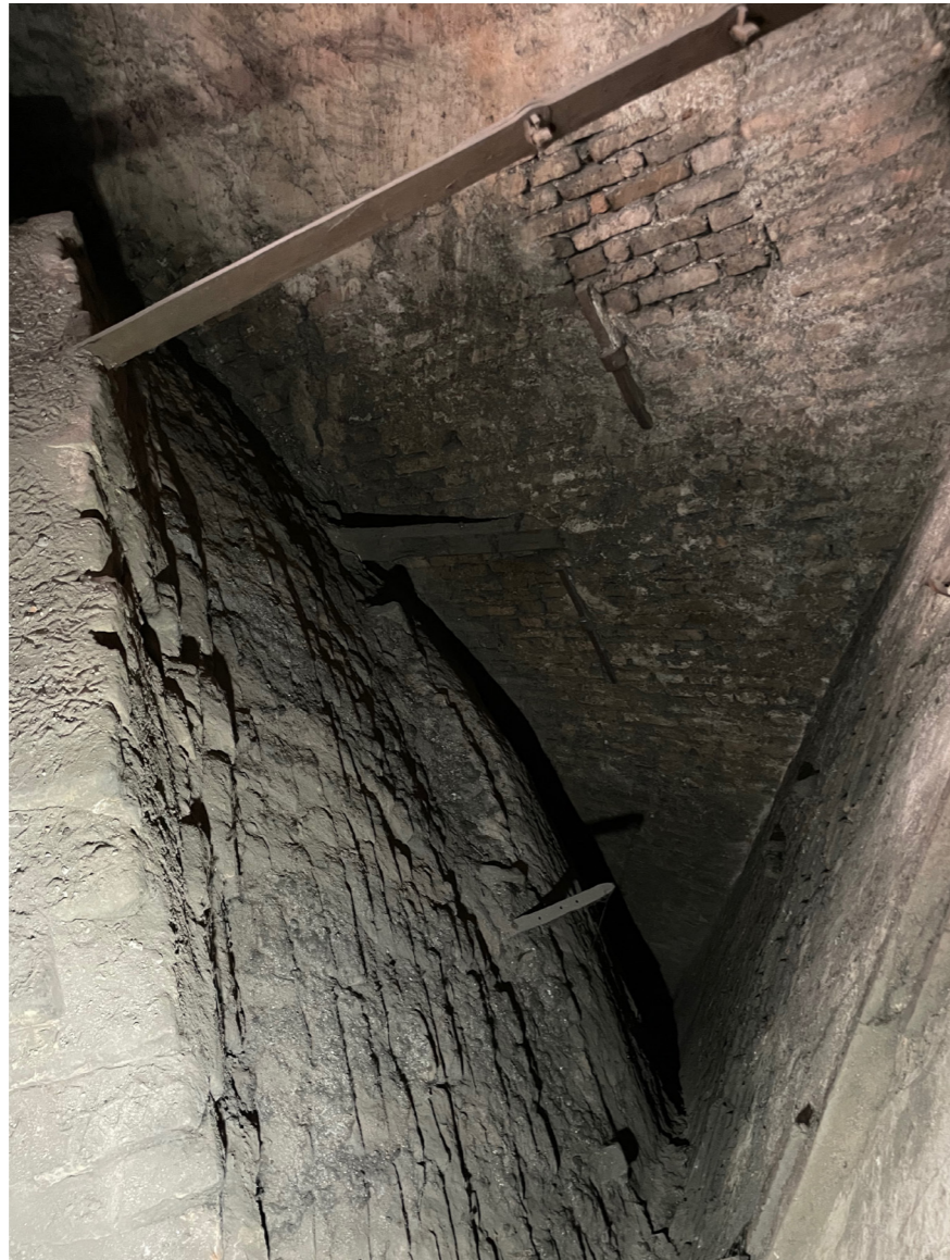
Figure 55 –The thin walls under the arconi resting on the pendentive extrados. Photography by Edoardo Piccoli, 2024.
