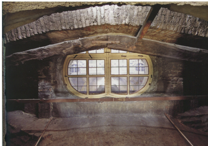
Figure 36 –The disconnected of the crown of the arcone and Chiave della Cupola . From Franco Rosso, Guarino Guarini , 2006. Photography by Giuseppe Dell'Aquila.
