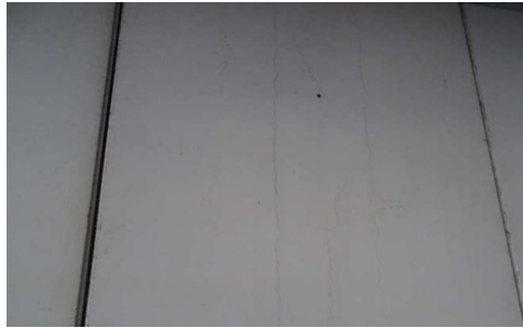
Figure 52 vertical cracks
