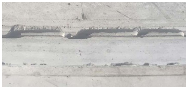
Figure 13 Example of hollows (SIG WG2, 2019)
