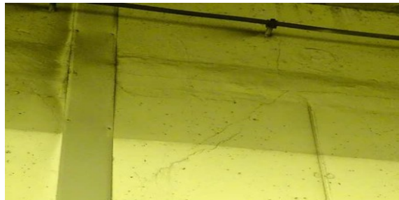
Figure 54 Diagonal crack
