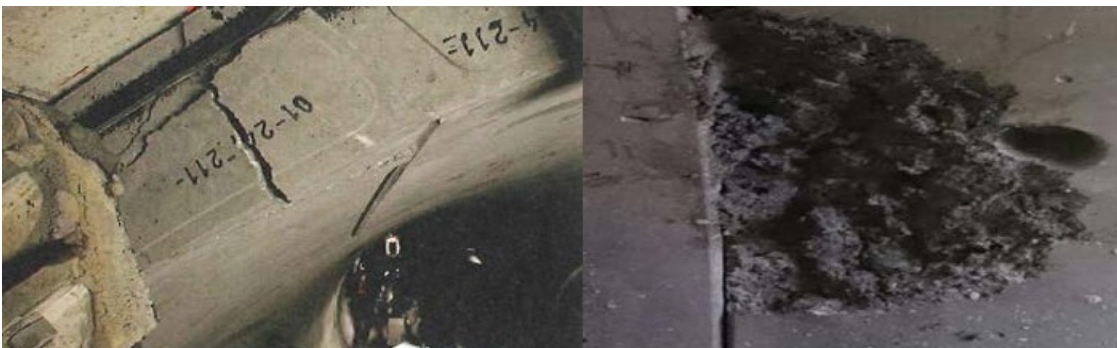
Figure 29 chippings in the corners (SIG WG2, 2019)
