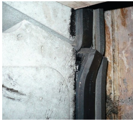
Figure 17 Expulsion of gasket from one side SIG WG2, 2019)
