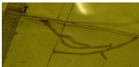
Figure 55 curvilinear cracks
