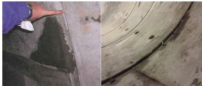
Figure 23 from left offset, from right a gap (SIG WG2, 2019)
