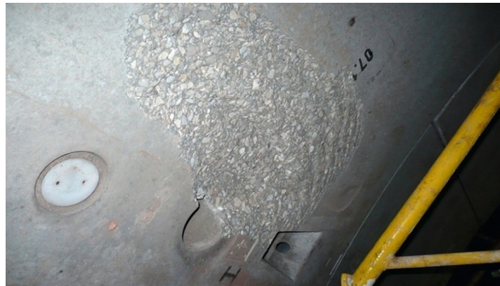
Figure 14 Exposed Aggregates (SIG WG2, 2019)
