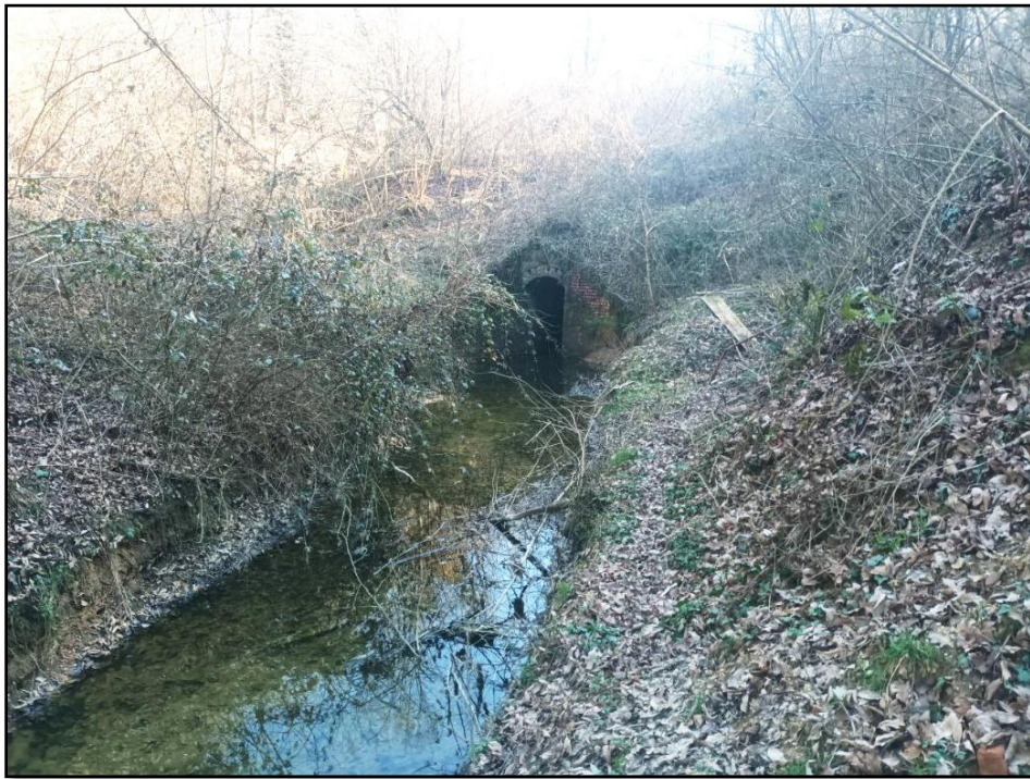
Photo 4: Entrance of the tunnel
