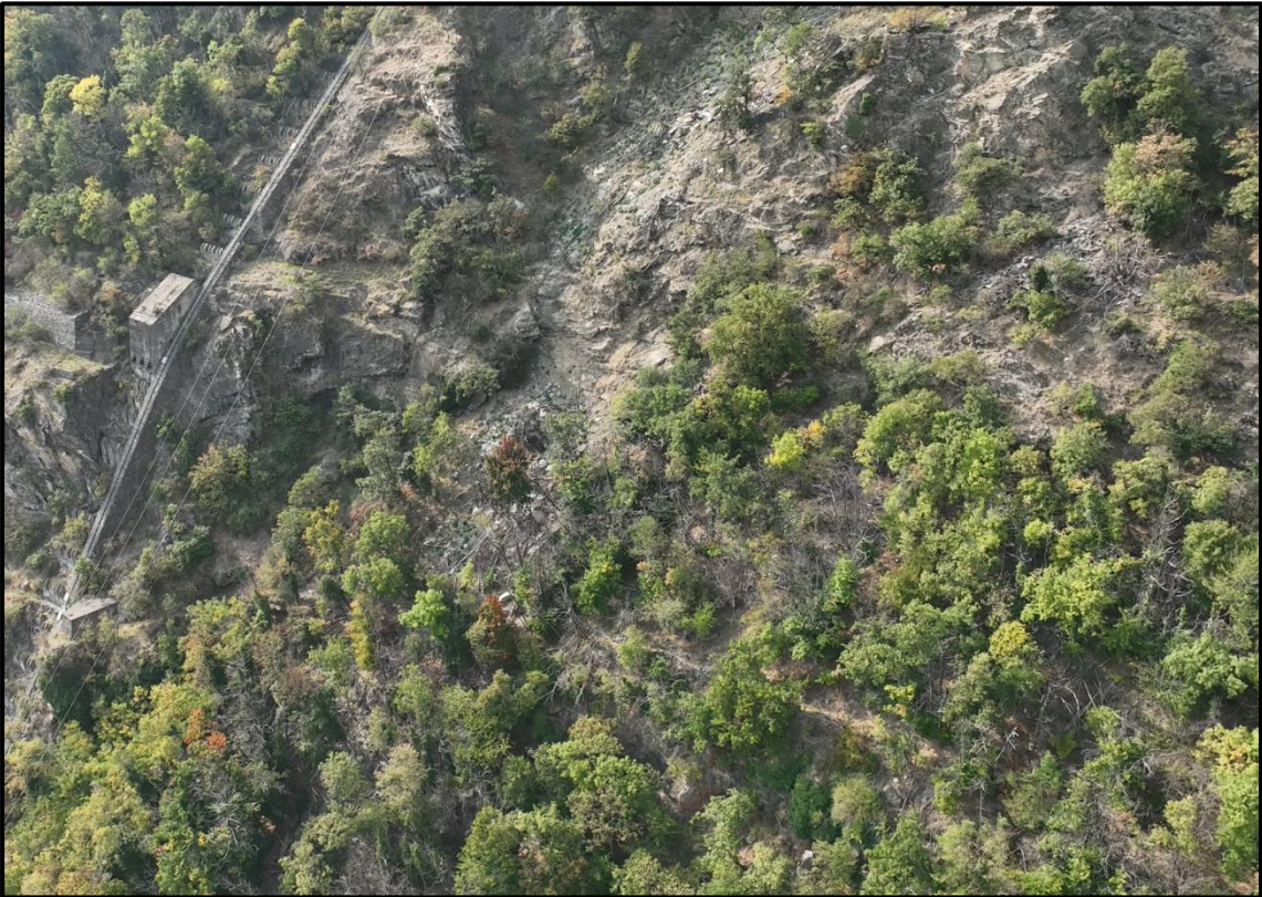
Figure 7.17 - Aerial view of the zone below rock wall No.2.
