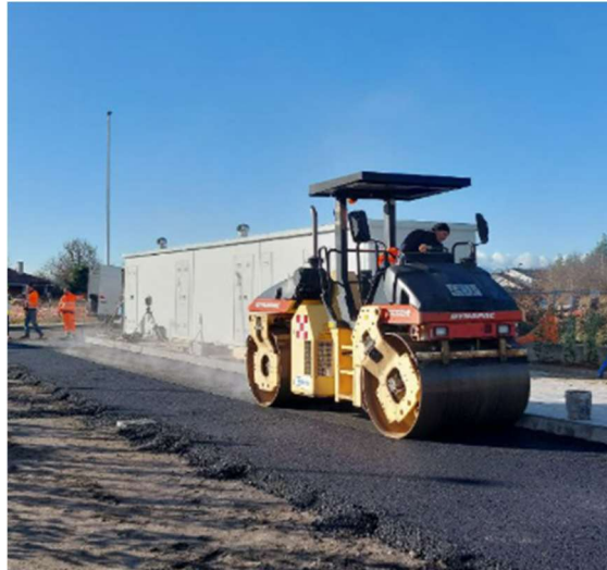
Figure 34 Field observation of asphalt laying operation
