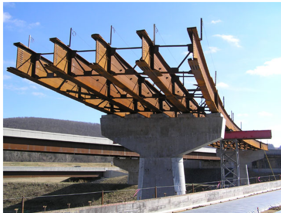
Figure 2.2. Construction of a Girder Bridge [11]
