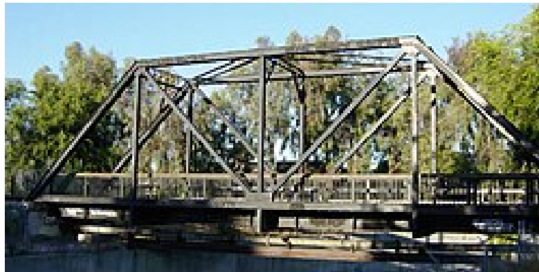
Figure 2.6. A truss bridge converted to pedestrian use and pipeline support [15]
