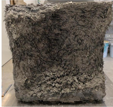
Figure 4-7: FRC specimen after fire exposure.
