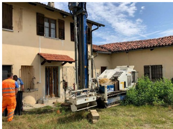
Figure 4.2: Second survey position
