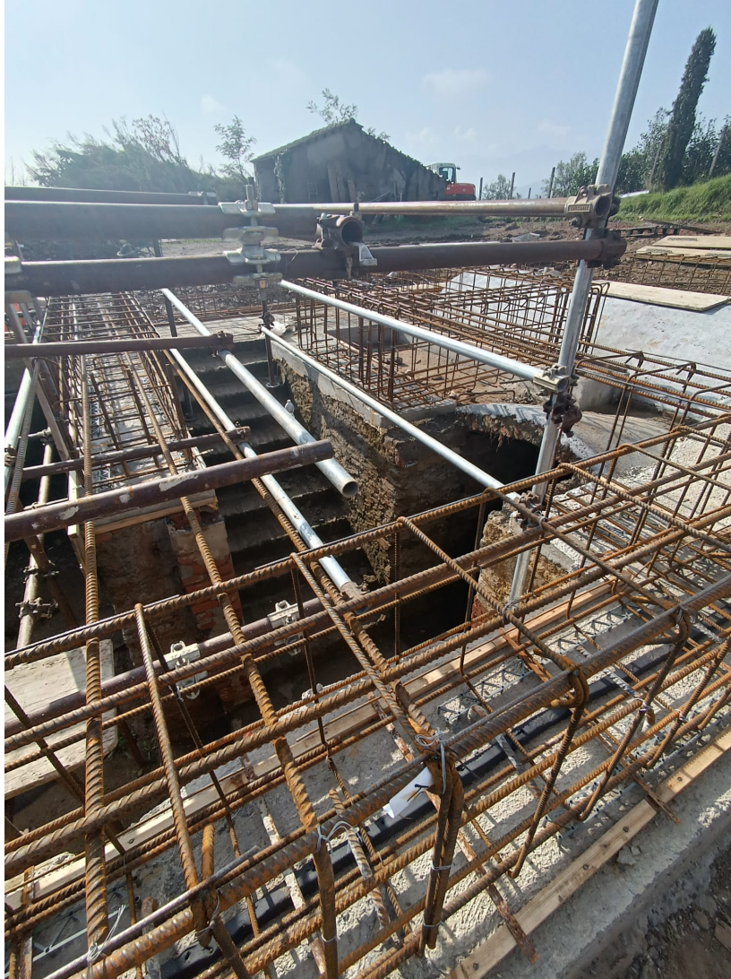
Figure 4.6: Basement roof slab
