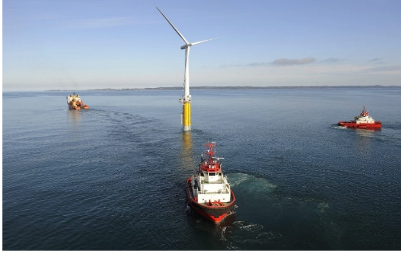
Figure 45: Tugboat towing a floating offshore wind turbine platform to the installation site.
