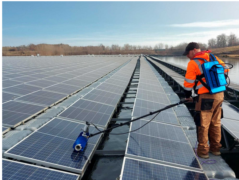
Figure 5.11: Illustration of a FPV cleaning (source [46]).
