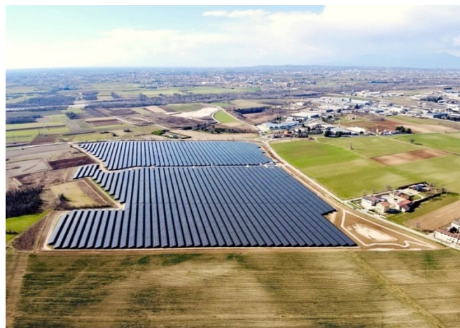
Figure 7: A 42 MW p utility-scale ground mounted PV system located near Udine, Italy [9]
