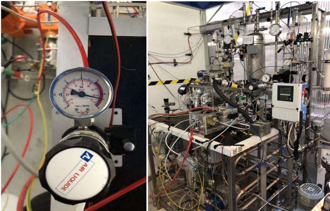
Figure 38 left: Air Pressure Regulator – right: assembled Baltic Fuel Cells to the test bench.
