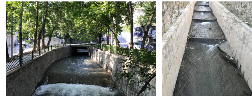
Fig. 3.53 - Darband: canale in cemento, tratti rettificati e soglie a gradoni; attraversamento tombato / Darband: concrete channel, straightened reaches and step-weirs; culverted crossing
