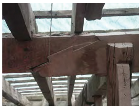
Figure 2.1.2.7 - Cutting and Displacement Technique: Overlapping New Piece for Extra Length
