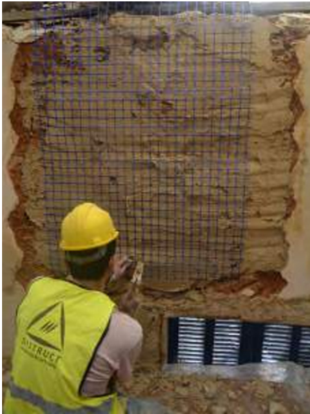
Figure 2.1.2.3 - IP Cracks Stitching Technique: Structural mesh installation (Right)
