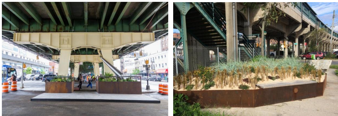
Left: Ground planters in Sunset Park, Brooklyn, collect rainwater through cone-shaped downpipes Right: The "Dune Landscape" planters in Rockaway, Queens, collect rainwater from the nearby elevated subway line (Rockaway Beach Union)
