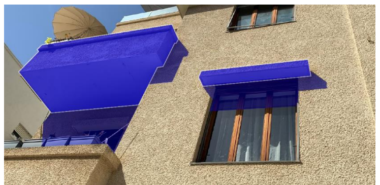
⬆ Fig.10 - Sheinkin St 55A, example of international style building with balconies and minimal brise-soleil extrusion with their shadowing surface (marked in blue), enhancing the protection from direct sun in the warm climate. Source: Photo by the author, September 12, 2024.
