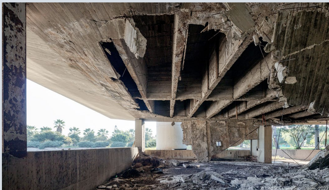
Figure 60. Photo of the collapsing ceiling of the underside of the OAT.
