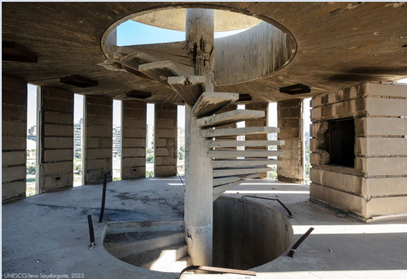
Figure 62. Interior photograph of the 3rd level of the tower (restaurant). Notice the deterioration of the central column.
