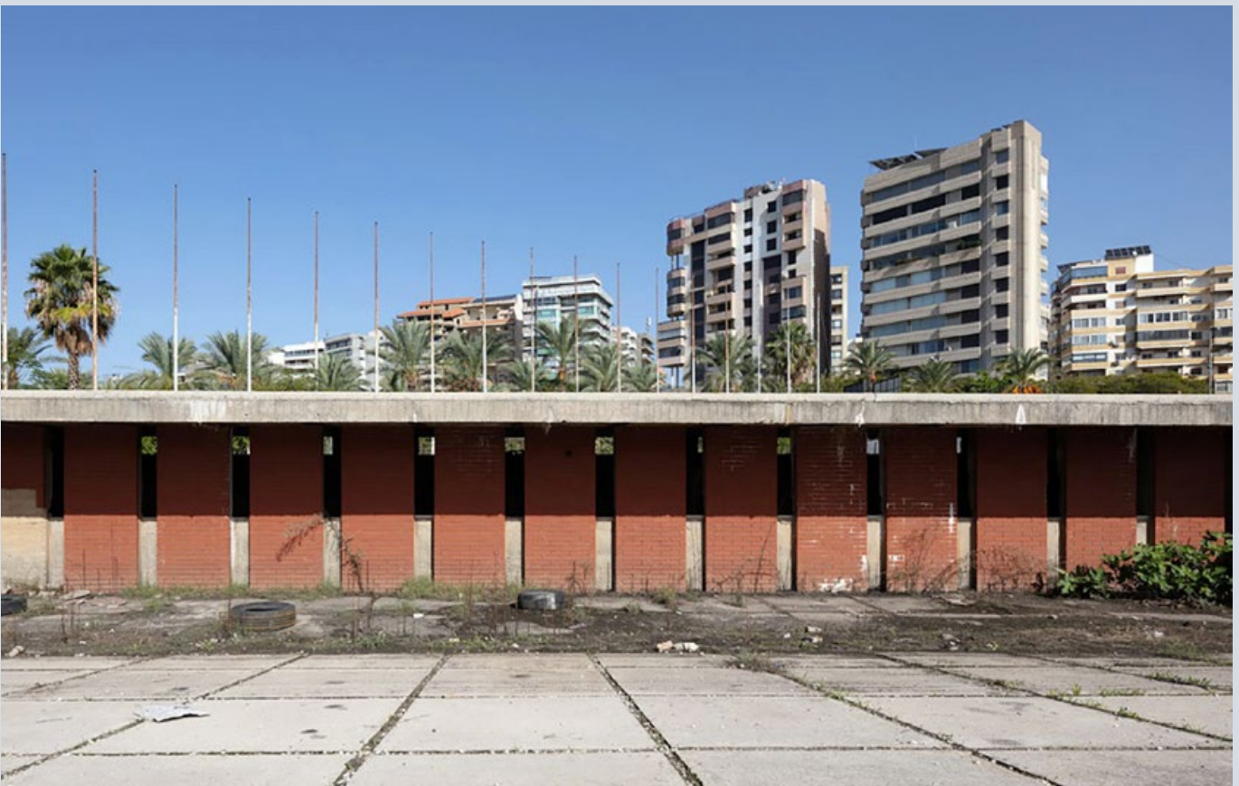
Figure 44. View of the main façade of the ticket booth. Notice the trace of water at the front.
