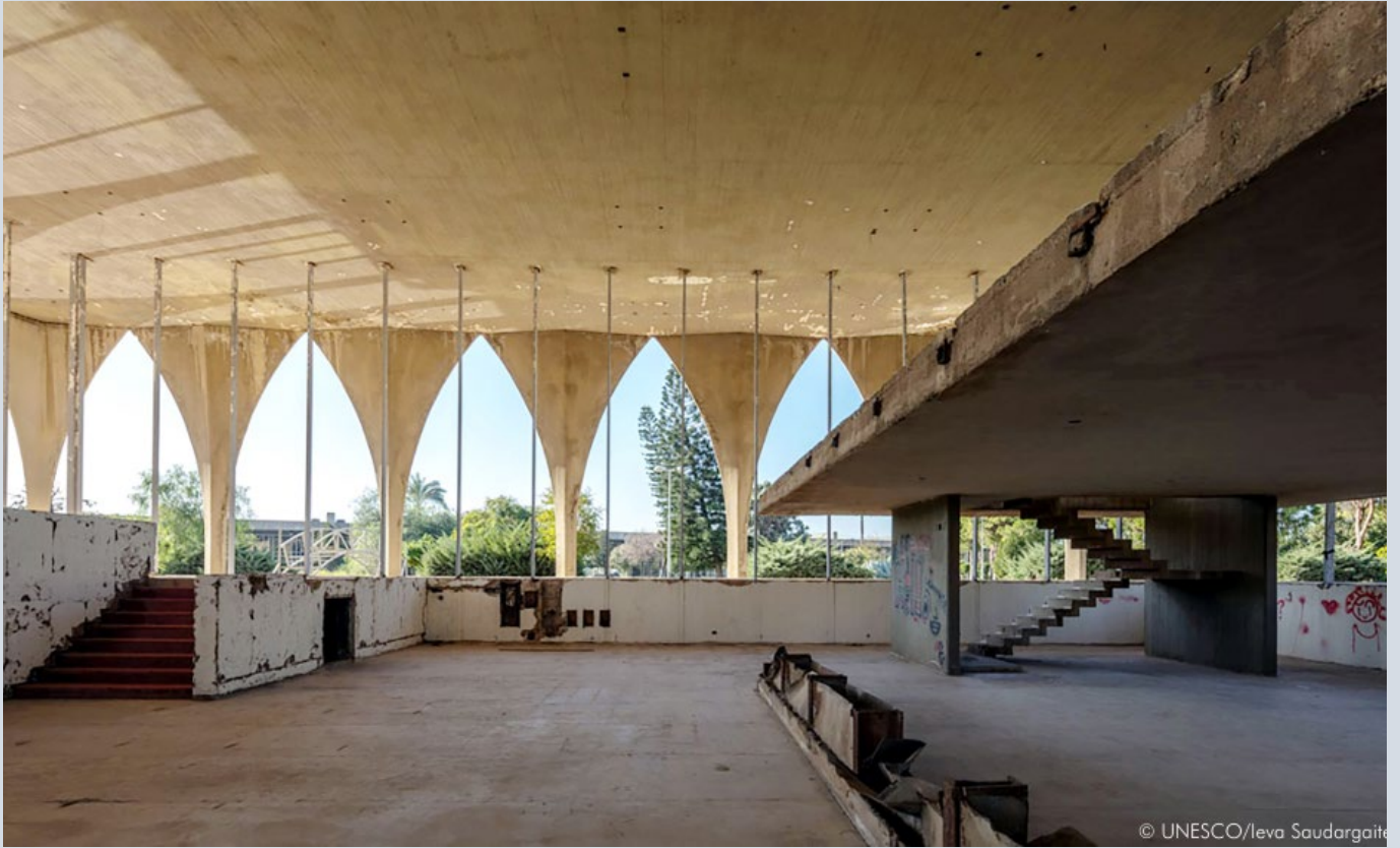
Figure 51. Interior of the Lebanon pavilion stripped from its linoleum tiles and white marble.
