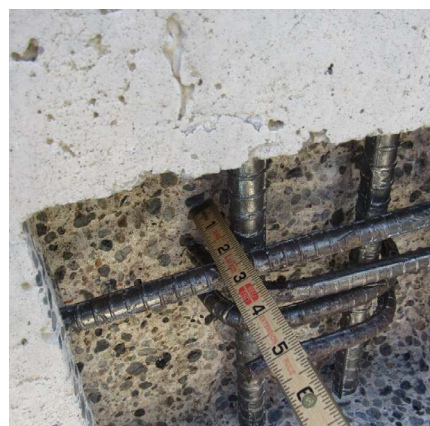
fig. 23. Removal of concrete beyond the reinforcement to allow for removal of corrosion and for proper bonding with the replacement concrete. Photo Ann Harrer and Paul Gaudette.
