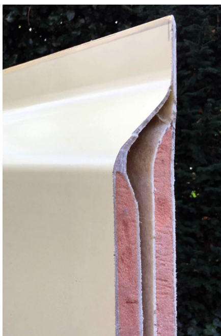
fig. 31. A section through a Herman Miller Factory facade panel, showing the two GRP sandwich panels that together form the facade. Photo R. Loader.
