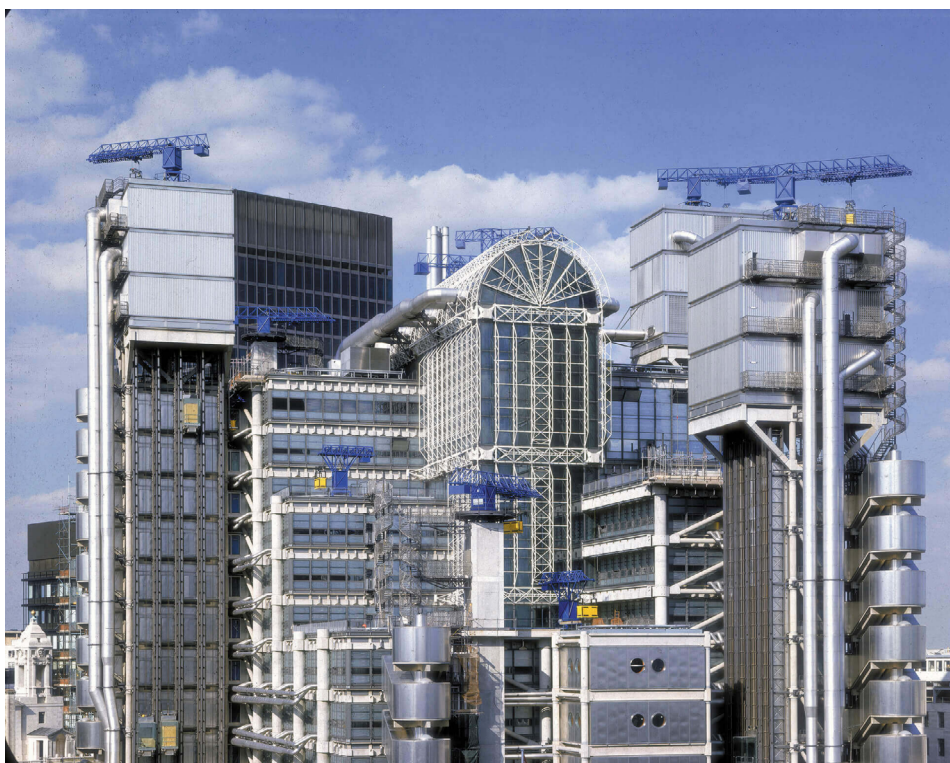
fig. 12. Lloyd's of London (Richard Rogers Partnership, 1986). The steel sandwich panels are used in the service towers. Photo RSHP.
