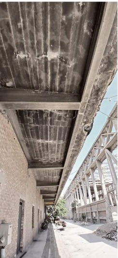
Figure X. Concrete slabs with wooden casting traces, Rey Cement Factory, Shahr-e Rey, Tehran. Photograph by the author, January 2024.
