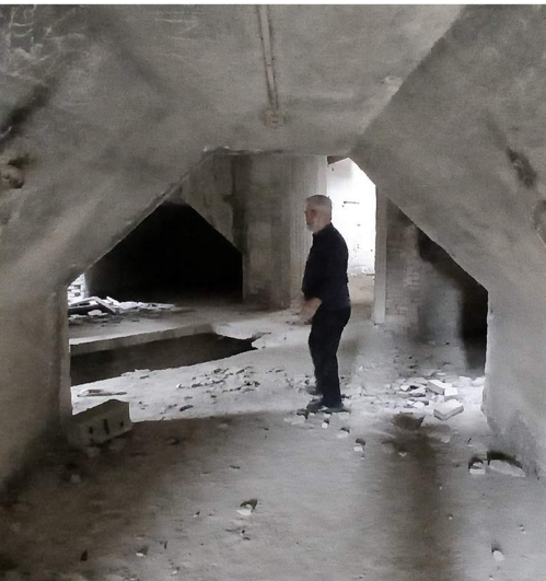
Figure X. Concrete bearing walls of the silos' underground passages, Rey Cement Factory, Shahr-e Rey, Tehran. Photograph by the author, January 2024.
