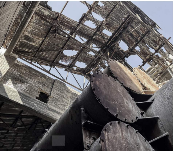
Figure X. Severe corrosion of the corrugated steel roof sheets of the 100-ton kiln building, Rey Cement Factory, Shahr-e Rey, Tehran. Photograph by Mostafa Roudaki, published by Mizan News Agency, n.d. https://www.bultannews.com/
