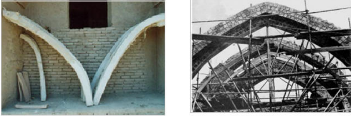
Fig. 67 construction method of the mold, reference: author and [73].
