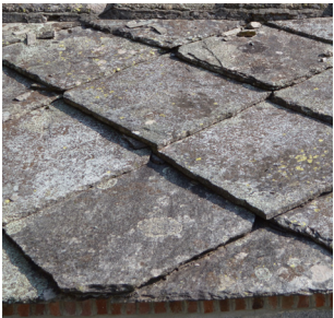
Local stone roof cut in Lose
