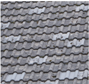
Roof with Marseillais tiles
