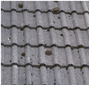
Roof with Marseillais tiles
