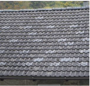
Roof with Marseillais tiles
