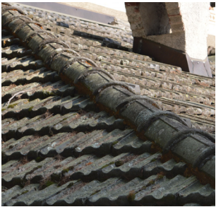
Roof with Marseillais tiles
