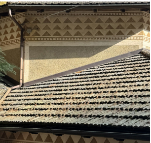
Roof with Marseillais tiles
