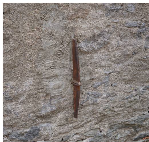
Reinforcement chain and tie rods. By Salvatore Tartaglia
