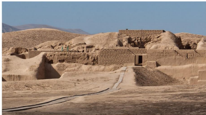
Fig. 14 Protective intervention methods: ground paving and brick addition
