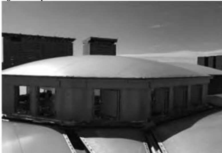
Figure8. Top Natural Ventilation Core
