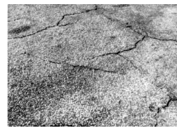
Block cracking
