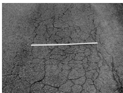
Alligator cracking
