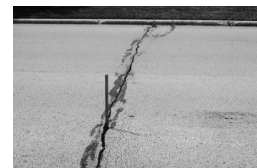
Transverse cracking
