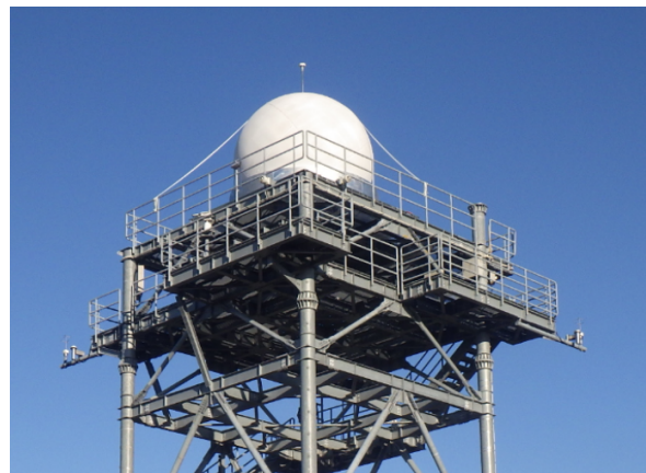
Figure 4.2: MP-PAWR radome installed in Saitama University (source: [23])
