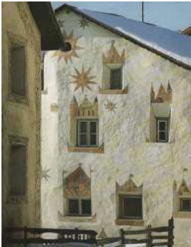
An example of Engadin House in Ardez. The volume, with its deep windows, is characterized by coloured Sgraffito decorations.
