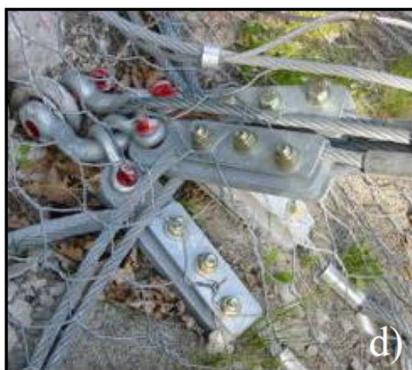
Figure 33: IGOR-SAFE brake system (Meccaferrri) (Marchelli M. , 2020)
