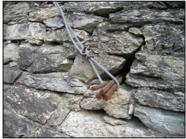
Figure 48: Inadequate anchor system (source: Marchelli M.)
