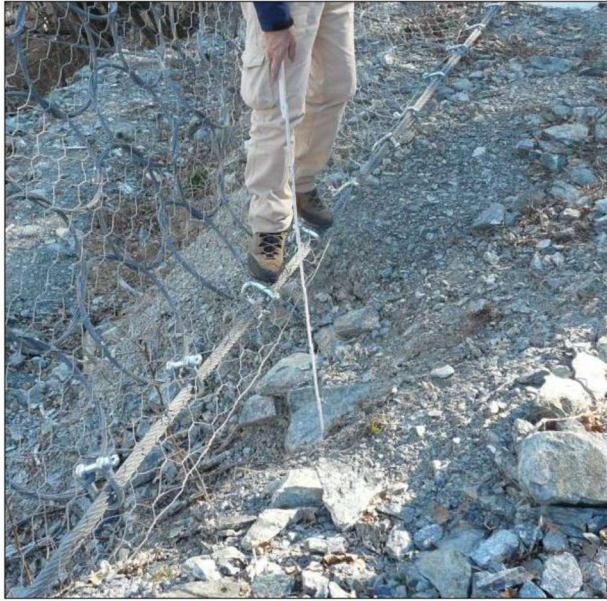
Figure 47: Presence of void at the bottom (source: Peila D.)
