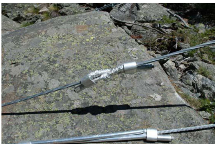
Figure 41: Mixed friction/plastic deformation string brake system: plastic deformation active (Meccaferrri, s.d.) and (RISP) (Marchelli M. , 2020)
