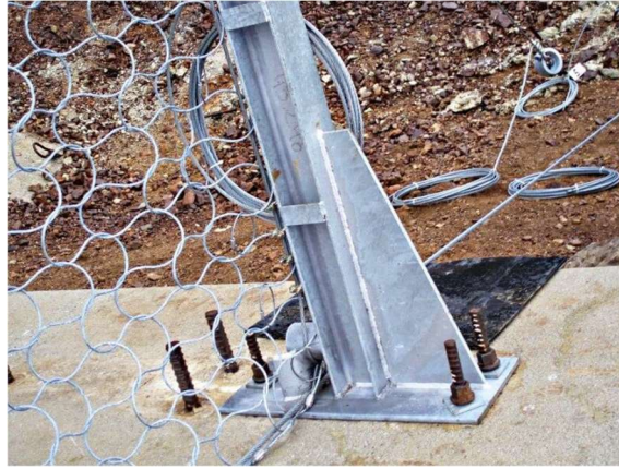
Figure 16: Fixed support (Marchelli M. , 2020)
