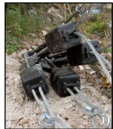
Figure 35: ISO-200 brake system (meccaferrri) (Marchelli M. , 2020)
