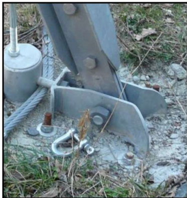
Figure 17: Mono-directional hinge (Marchelli M. , 2020)
