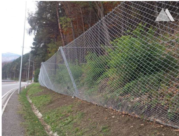
Figure 12: Rhomboidal net in exercise (Geobrugg, s.d.)
