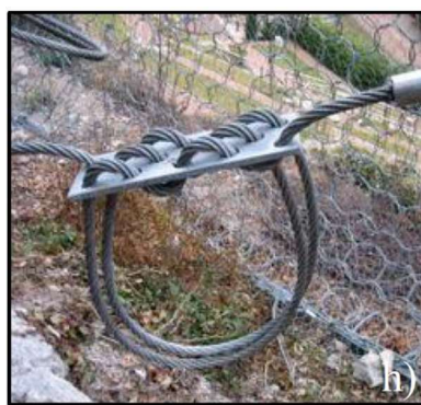
Figure 34: ISOFER-INCOFIL brake system (INCOFIL) (Marchelli M. , 2020)
