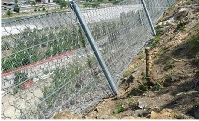
Figure 6: Rockfall barrier. (Geobruigg, s.d.)
