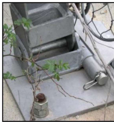
Figure 18: Bi-directional hinge (Marchelli M. , 2020)
