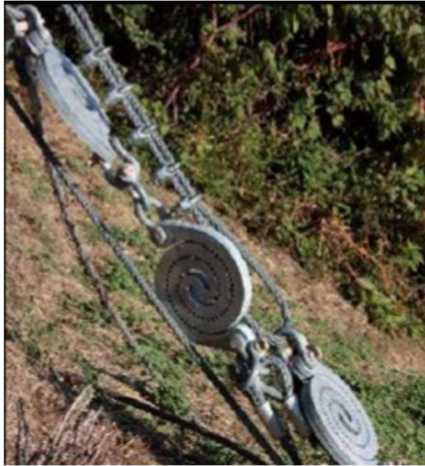
Figure 37: plastic deformation brake system: isodisk (PFEIFER) (Marchelli M. , 2020)
