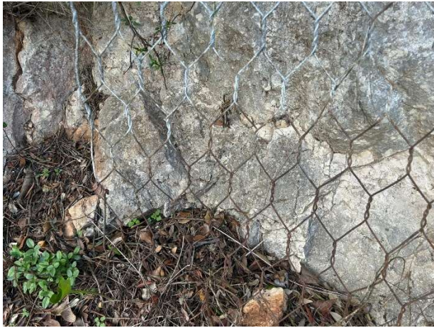
Figure 109: State of the wire mesh of element (c)
