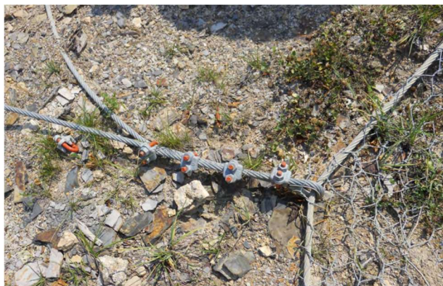
Figure 28: Loaded wire rope cable anchor (Ingram & Wagner, 2012)
