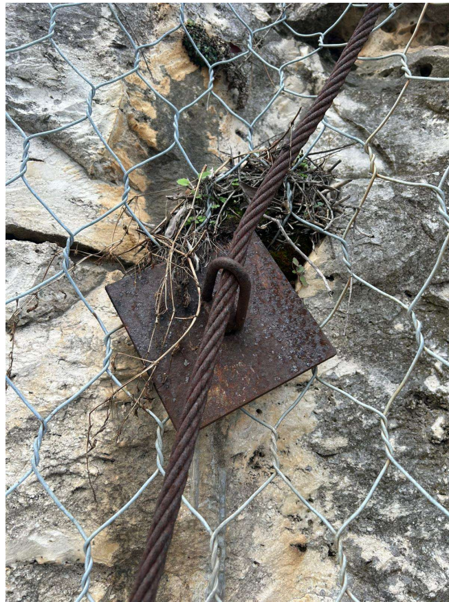
Figure 112: Anchor plate and anchor system of the element (d)
