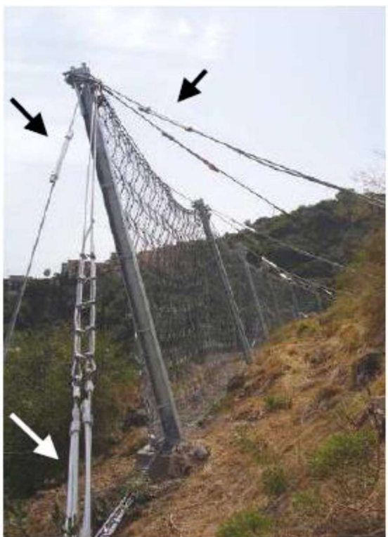
Figure 39: Mixed friction/plastic deformation: string brake system (Meccaferrri, s.d.) (Marchelli M. , 2020)
