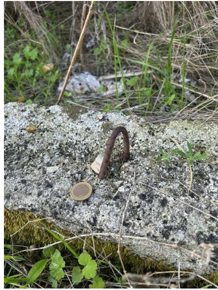
Figure 107: State of the anchor of the case (b)
