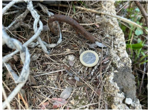
Figure 110: State of the anchor of the element (c)
