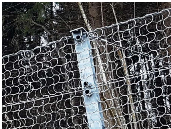
Figure 13: Omega net in exercise (Trumer Schutzbauten, s.d.)
