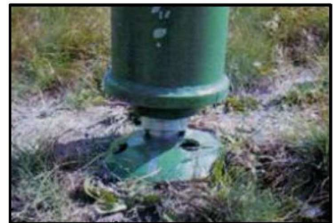
Figure 19: Spherical hinge (Marchelli M. , 2020)
