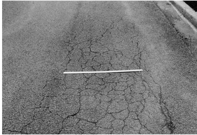
Figure 1.1.2 - Medium severity alligator cracking.
