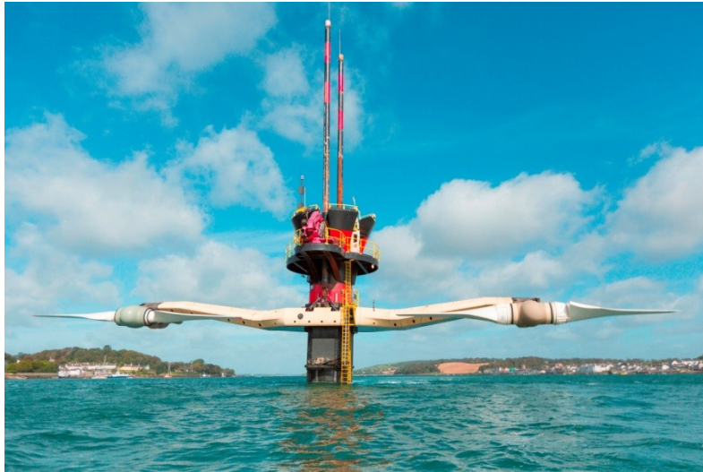
Figure 1.5: Seagen, 1.2 MW, monopile foundations. [5]
