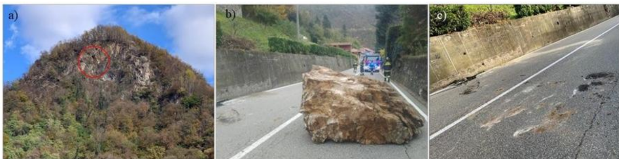
Figure 10. a) detachment niche located on the Barbavara castle rock slope; b) kinzigite rock block of about 3 \text{ m}^3 that detached in c) road damaged by the rock collapse[1]
