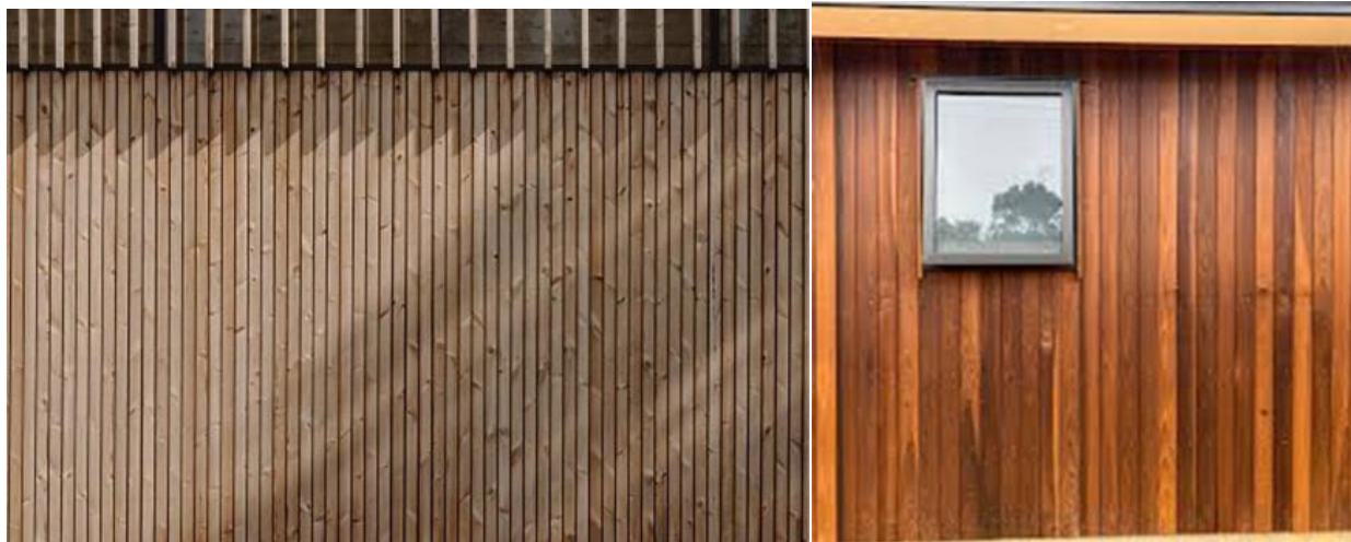
Figure 35– TMT wood panel
