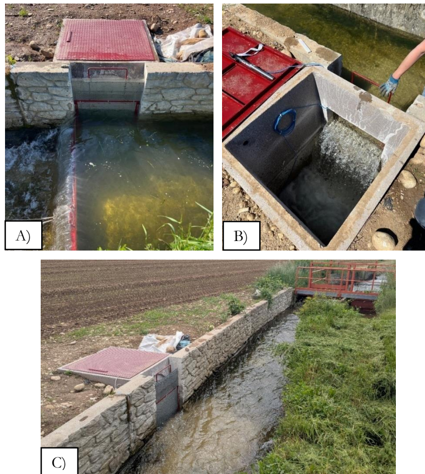
Figure 11. Photographs taken at Tetti Pesio MAR system: A) sluice gate connecting the channel to the collection chamber; B) collection chamber; C) irrigation channel integrated with the MAR structure.
