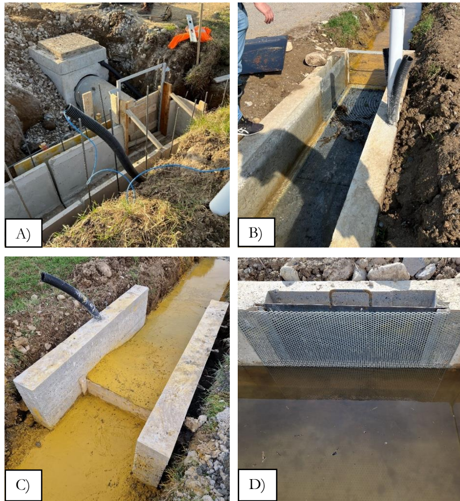
Figure 10. Photographs taken during construction works: A) pipe connection between the collection chamber and the concrete section of the channel; B) concrete section with the fine-mesh grid installed; C) one of the two broad-crested weirs; D) sluice gate that regulates the flow to the collection chamber.
