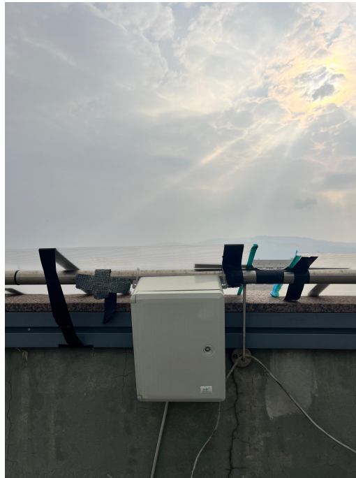
Figure 5.2: PoliTO6 placement on the roof
