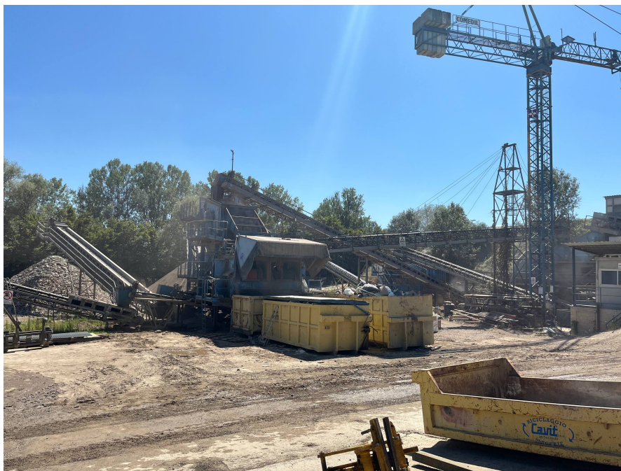
Figure 3.1: General view of the CDW recycling facility in Torino, Piedmont region
